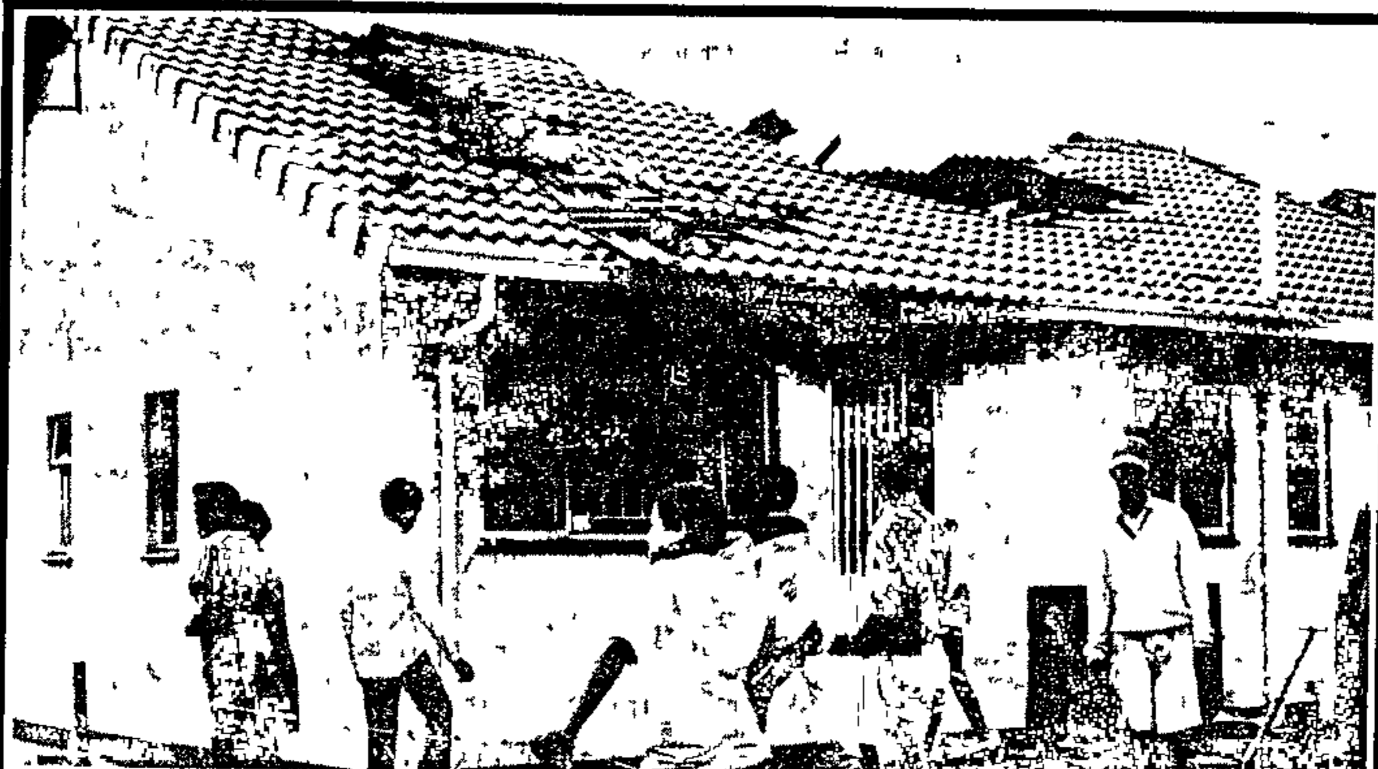
IF WE DON'T STAY HERE, NOBODY WILL Several houses in Ennerdale Extension 5, south of Johannesburg, went up in flames after families were evicted for not paying rent. People had complained to the Johannesburg City Council about cracked walls and leaking roofs and decided not to pay until their grievances were addressed. Evictions started on Tuesday
