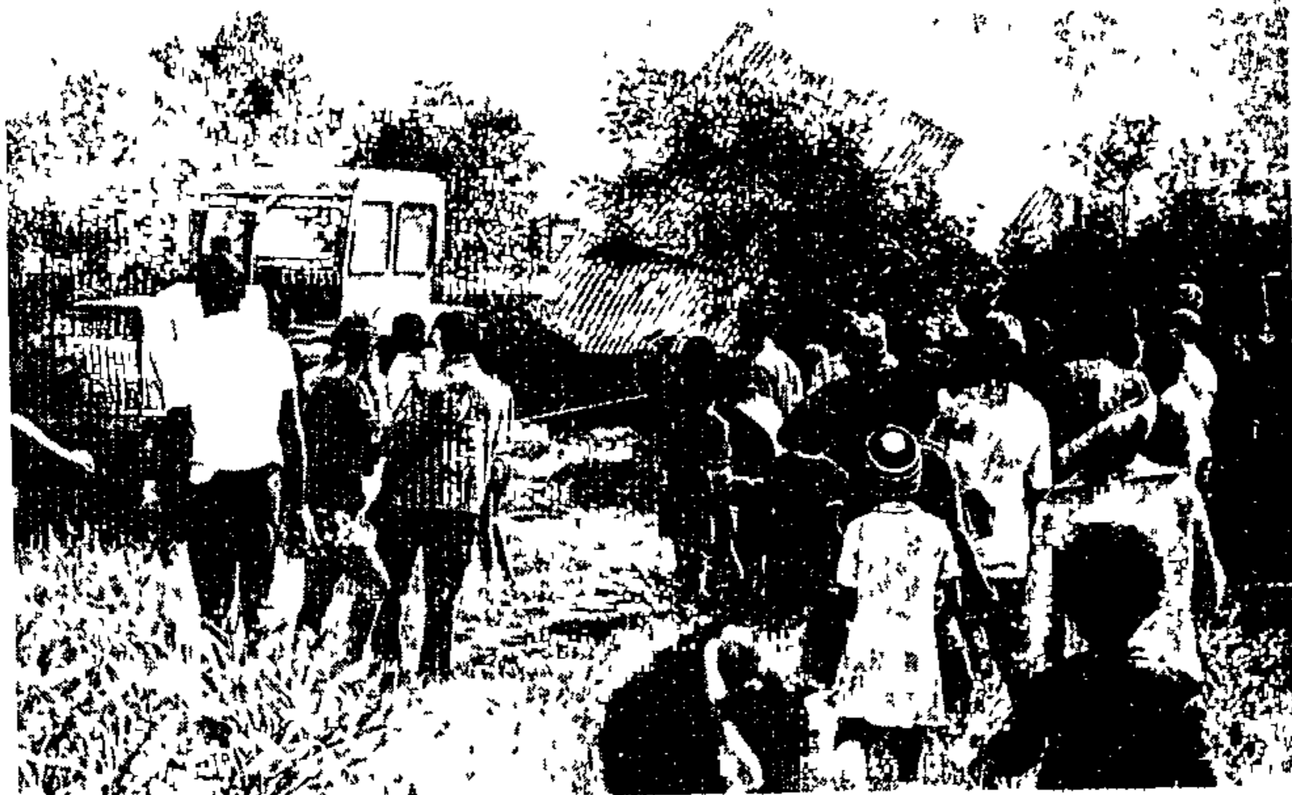
Love may be love . . . but not when the demolishers arrive
