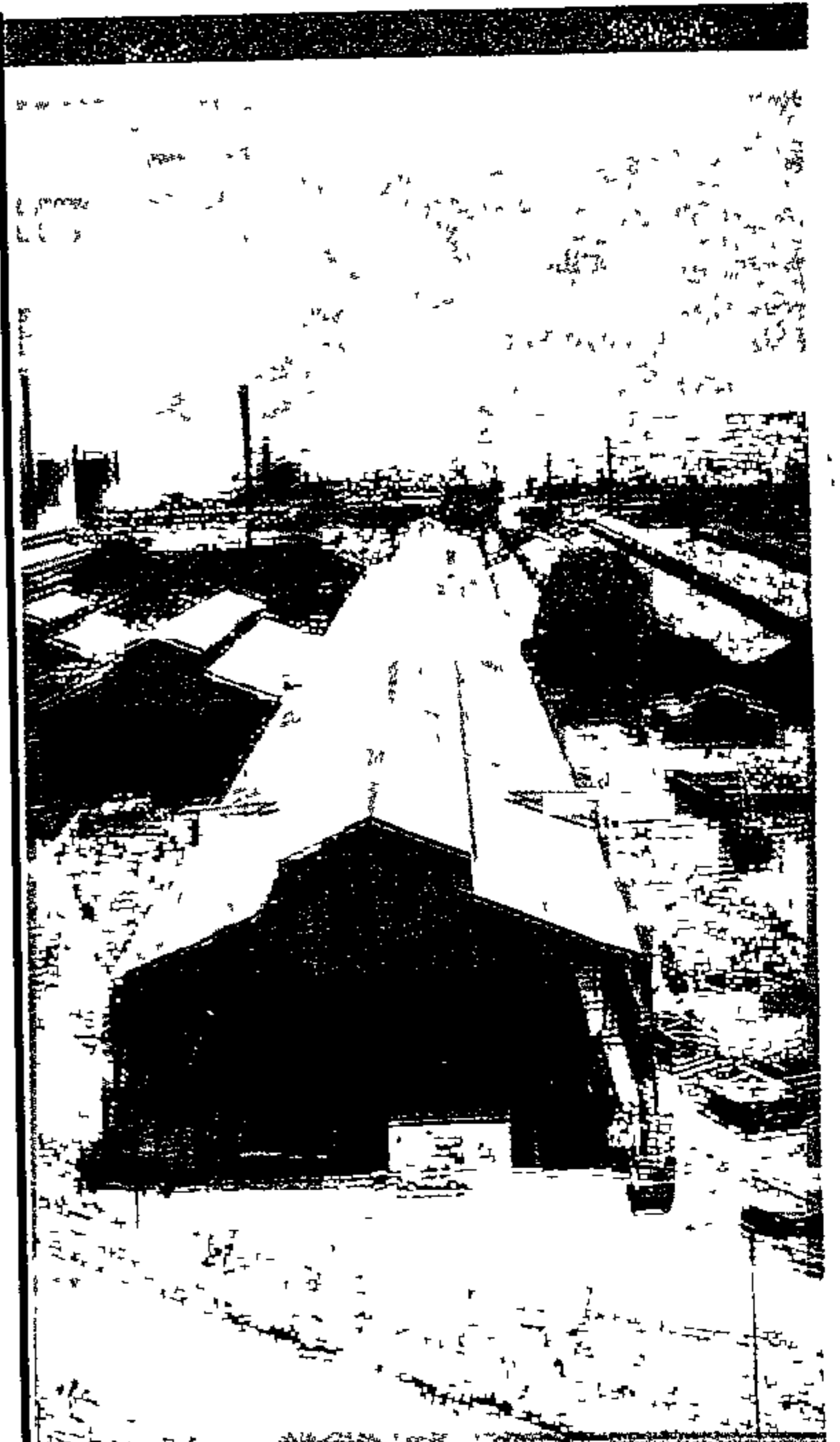
During the 40 years of its existence, the Iscor plant at Pretoria has grown from a small building standing in isolation on the bare veld to an enormous industrial complex as shown here.
