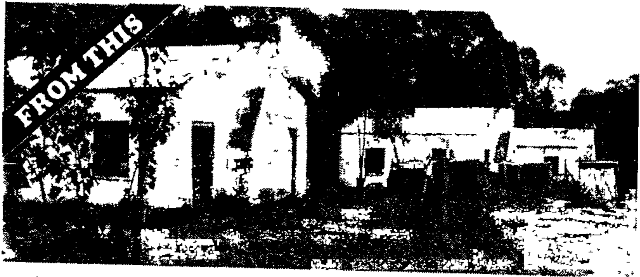
The cottages near the old power station which have to make way for industry
