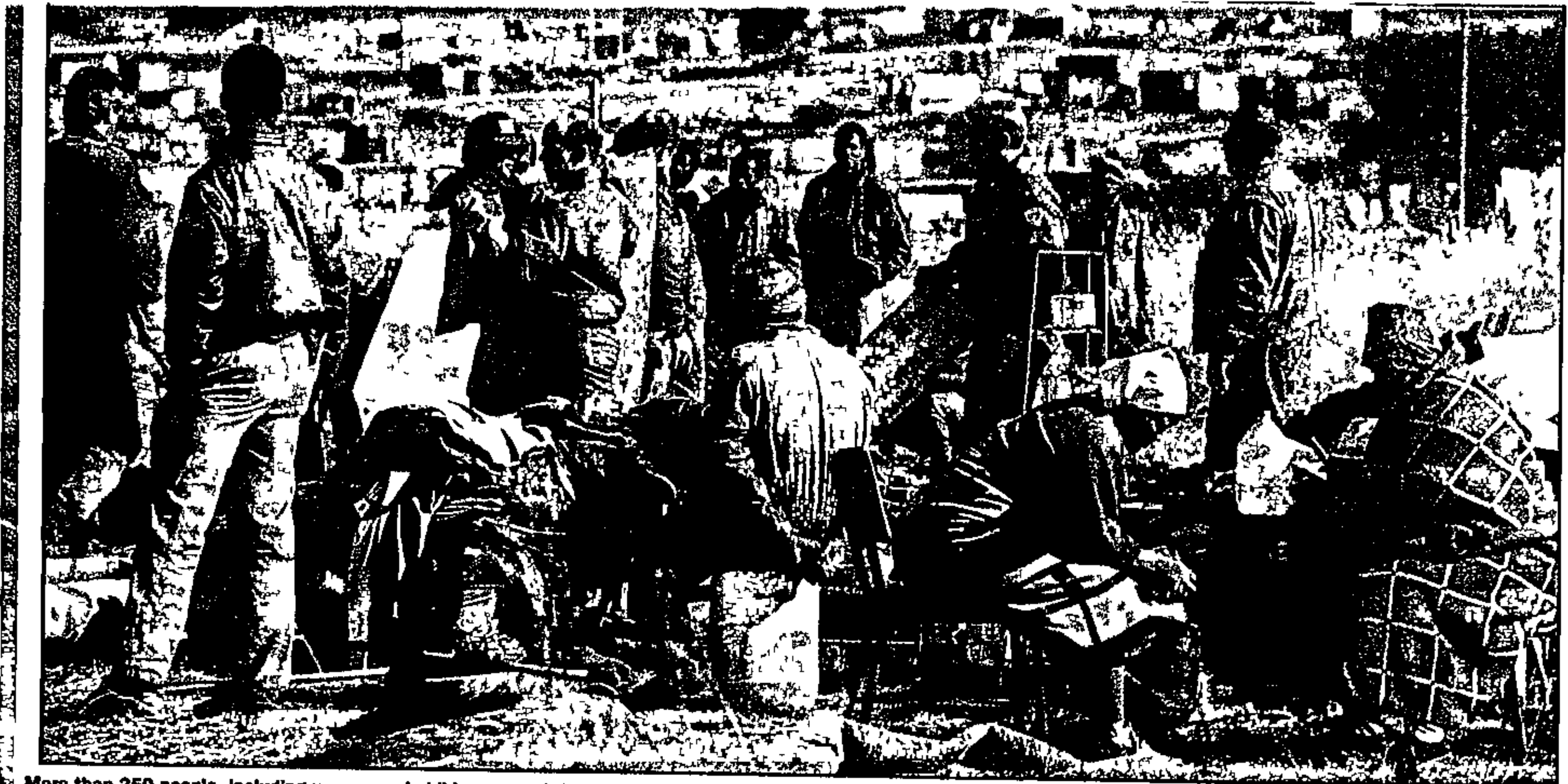
More than 250 people, including women and children, were left out in the cold after police and Johannesburg City Council officials demolished their shacks at Devland yesterday. A spokesman for the council accused the families of "land invasion" and said its security personnel had acted on "strict instructions" to demolish the shacks. PIC LEN KUMALO
