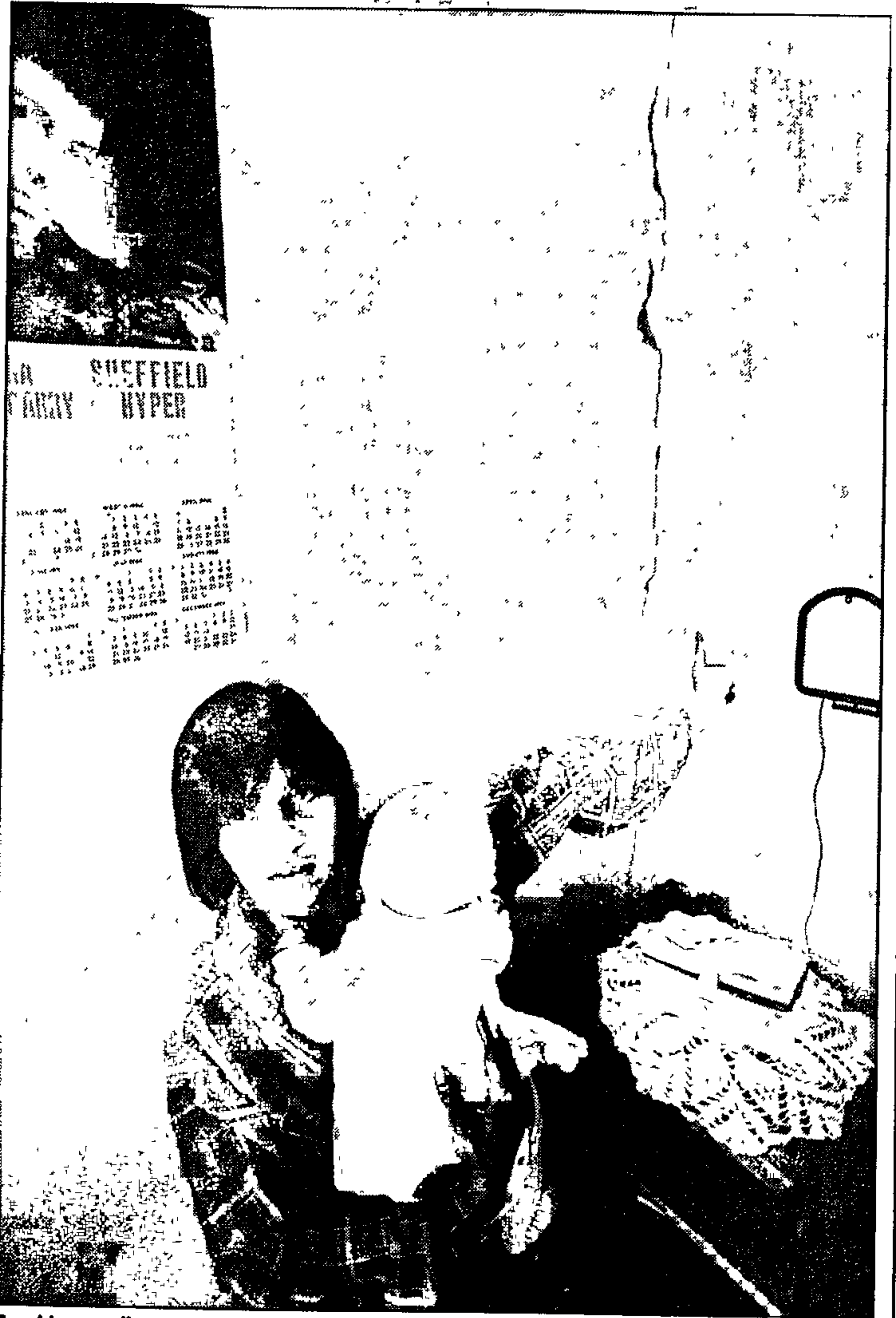
Cracking walls . . . Shanita Armugam had to cement the walls of her home three times this year and fears her home will fall apart in the coming heavy rains. She says the foundations of her home are faulty.
