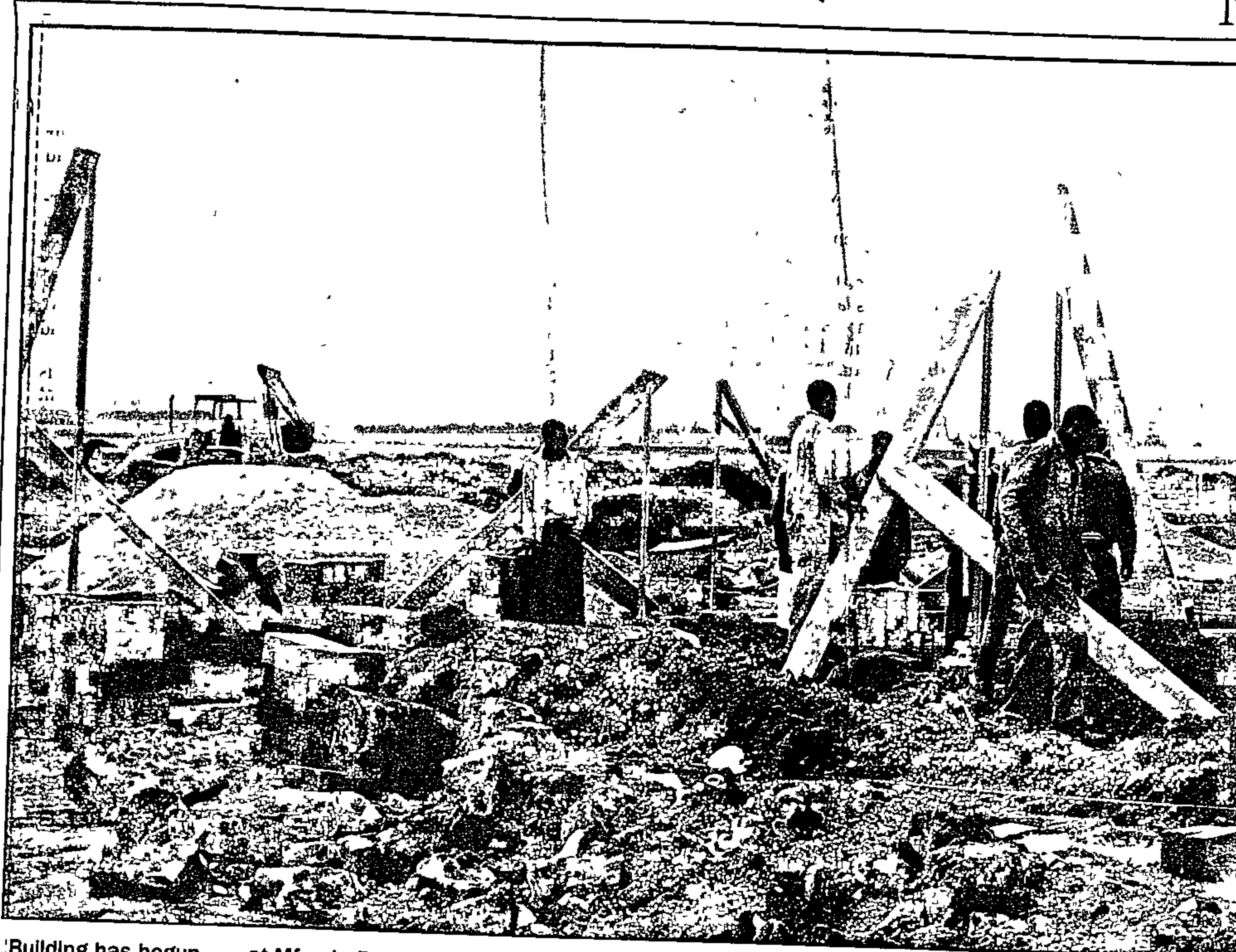
Building has begun . . . at Mfundo Park for the Star Homes Show 1991. An extra 14 showhouses will go on display. Picture. John Hogg
