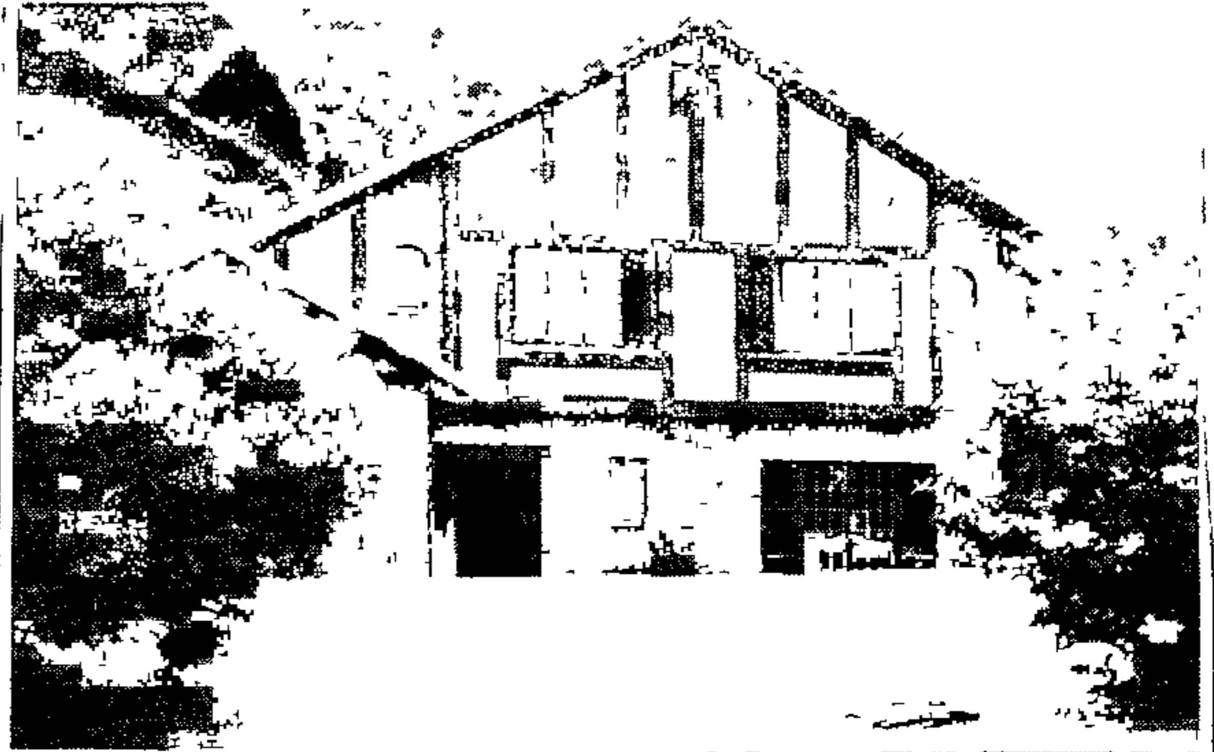
The R150 000 Port Shepstone house at the centre of a storm after the outgoing mayor, Mr Peter King, had apparently sold it to an Indian businessman. NIM 112/87
