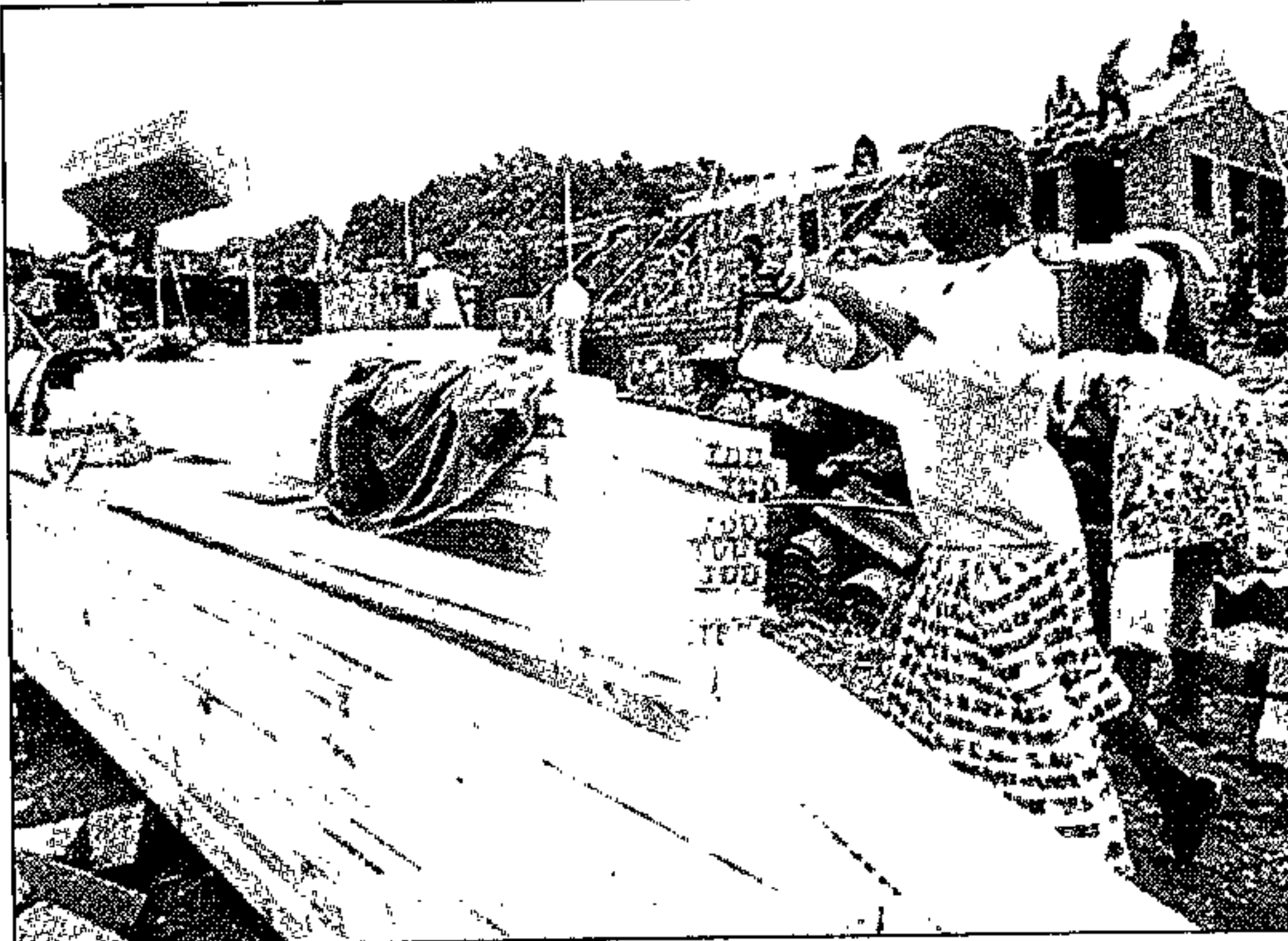
Building the future: An Mpumalanga woman works at building a house in the province that has seen substantial co-operation between the government and the private sector
