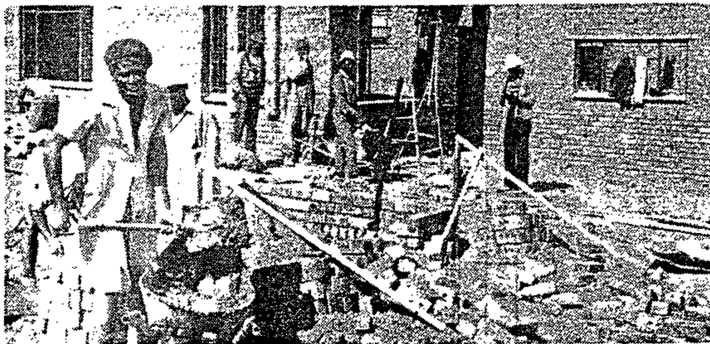
Builders putting up houses in the townships.
