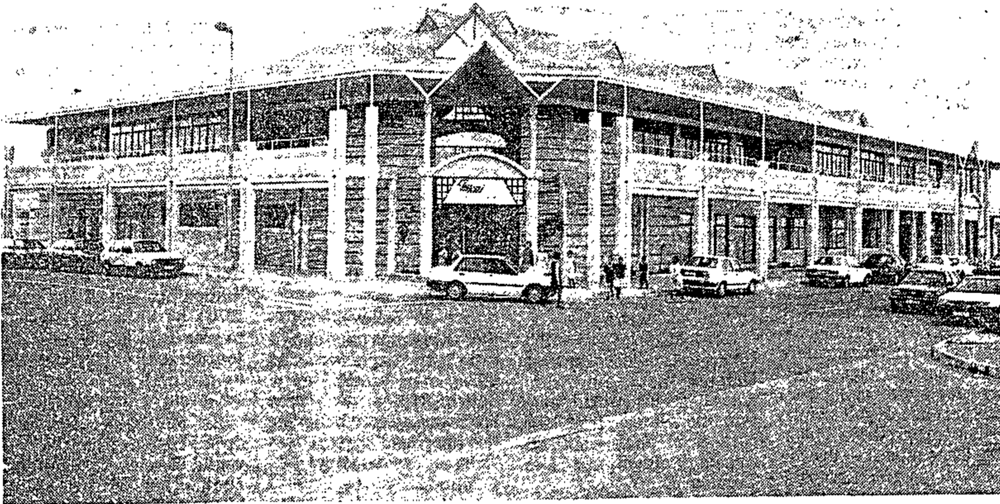
The Ciskei Building Society's new head office in Bisho, designed by Raymond Drake of Osmond Langa, is L-shaped and scaled to form a link between the CBD and an upmarket residential area. However, the building is large enough to allow for ample growth in the society's business and cater for the needs of a modern financial institution.
