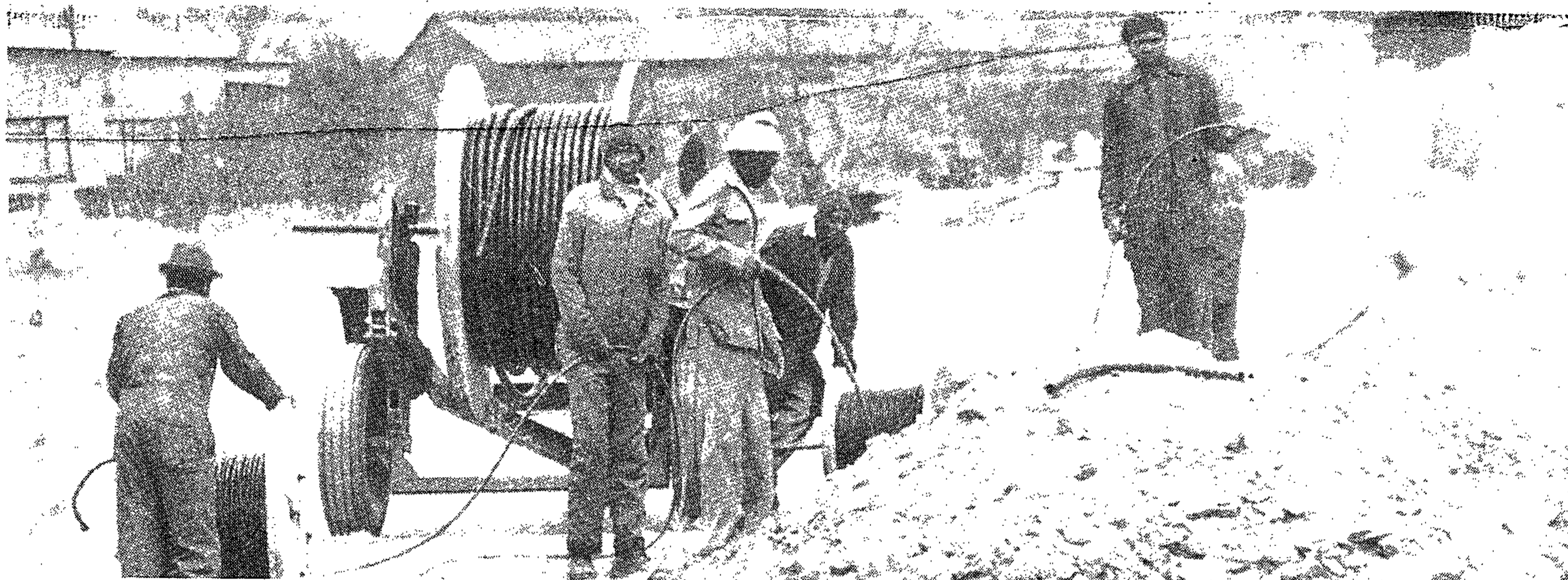
Workmen busy laying cables in one of the major electrification projects in the country. But still there are millions of South Africans who don't have electricity.
