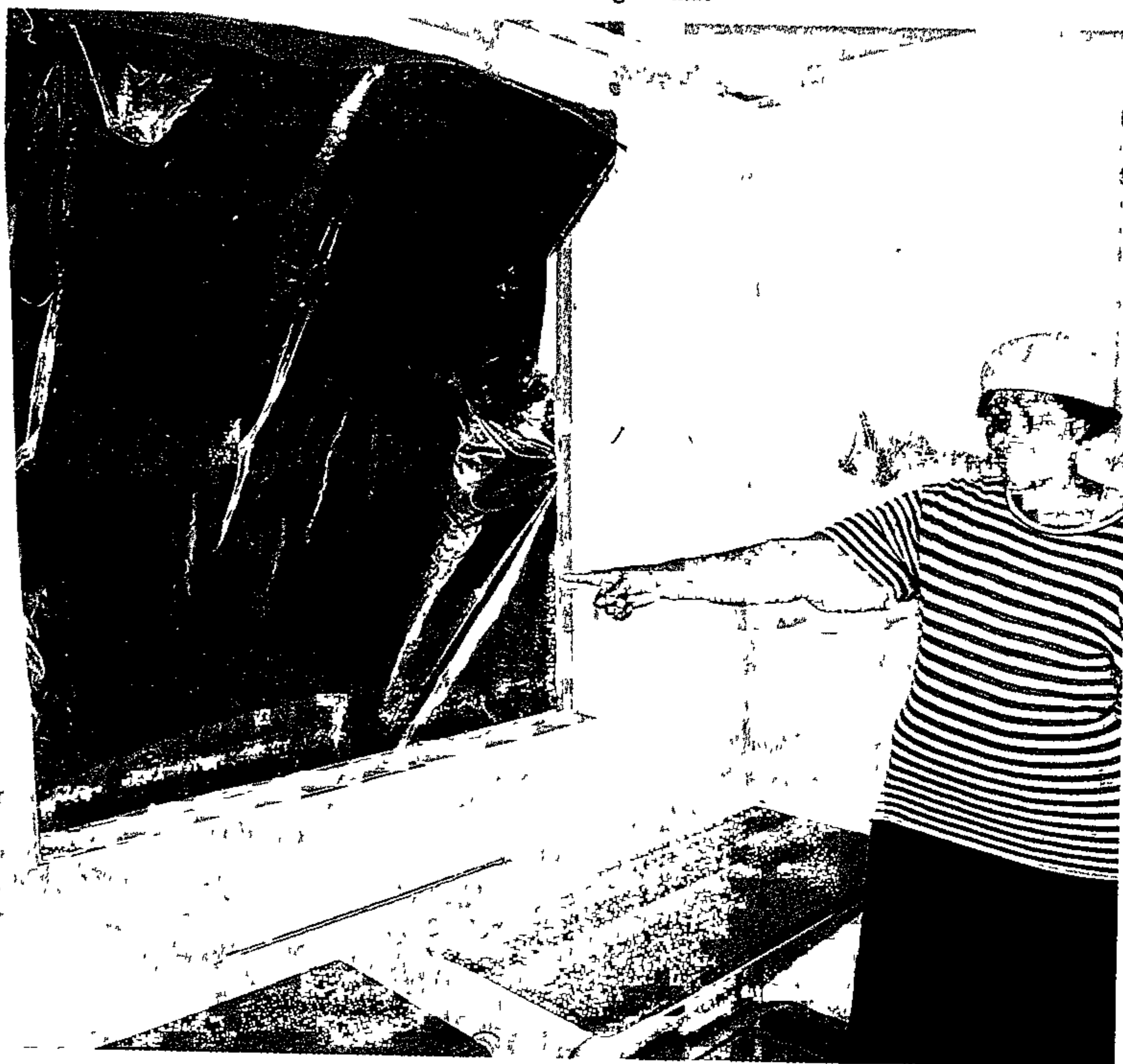
STRIFE DAMAGE: Driftsands Residents' Committee member Zoda Tika points to black plastic used to fill a window of the Driftsands crèche.
