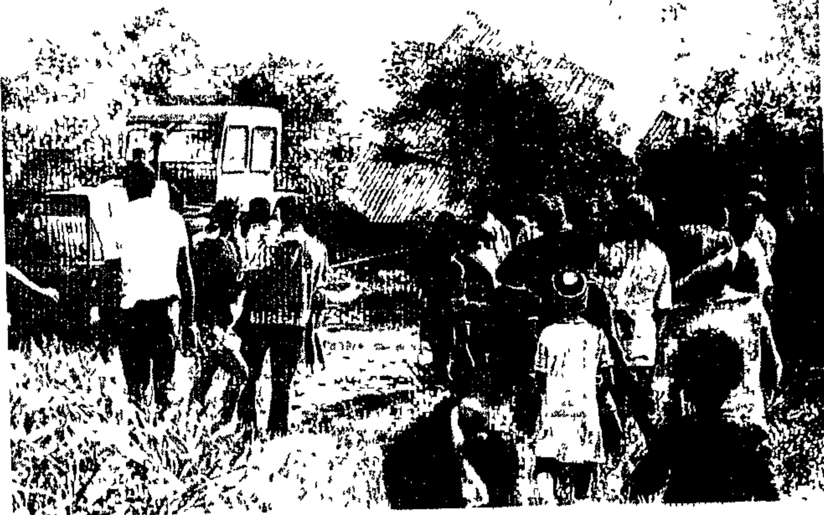
Love may be love . . . but not when the demolishers arrive
