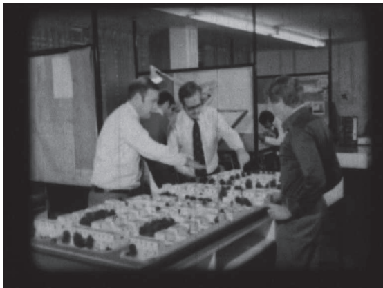
Fig. 2.35 City engineers over model project (1)
