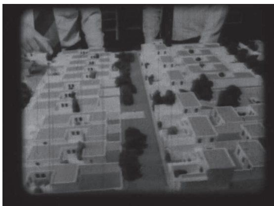
Fig. 2.36 City engineers over model project (2)
