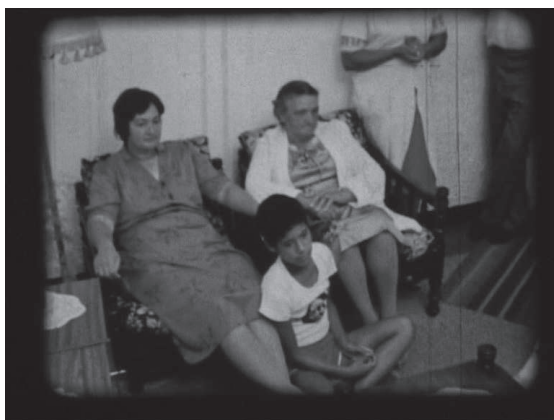
Fig. 2.33 Older housing schemes - Lounge (1)
