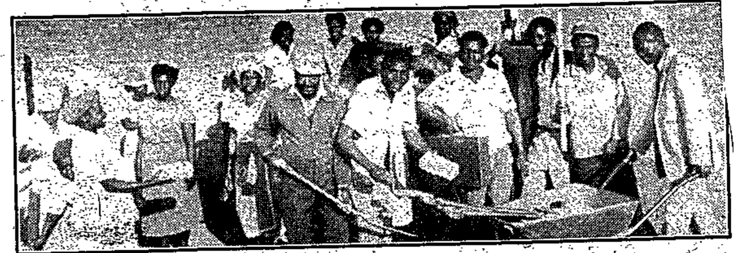
Workers at the Nzhelele Civic Centre.
