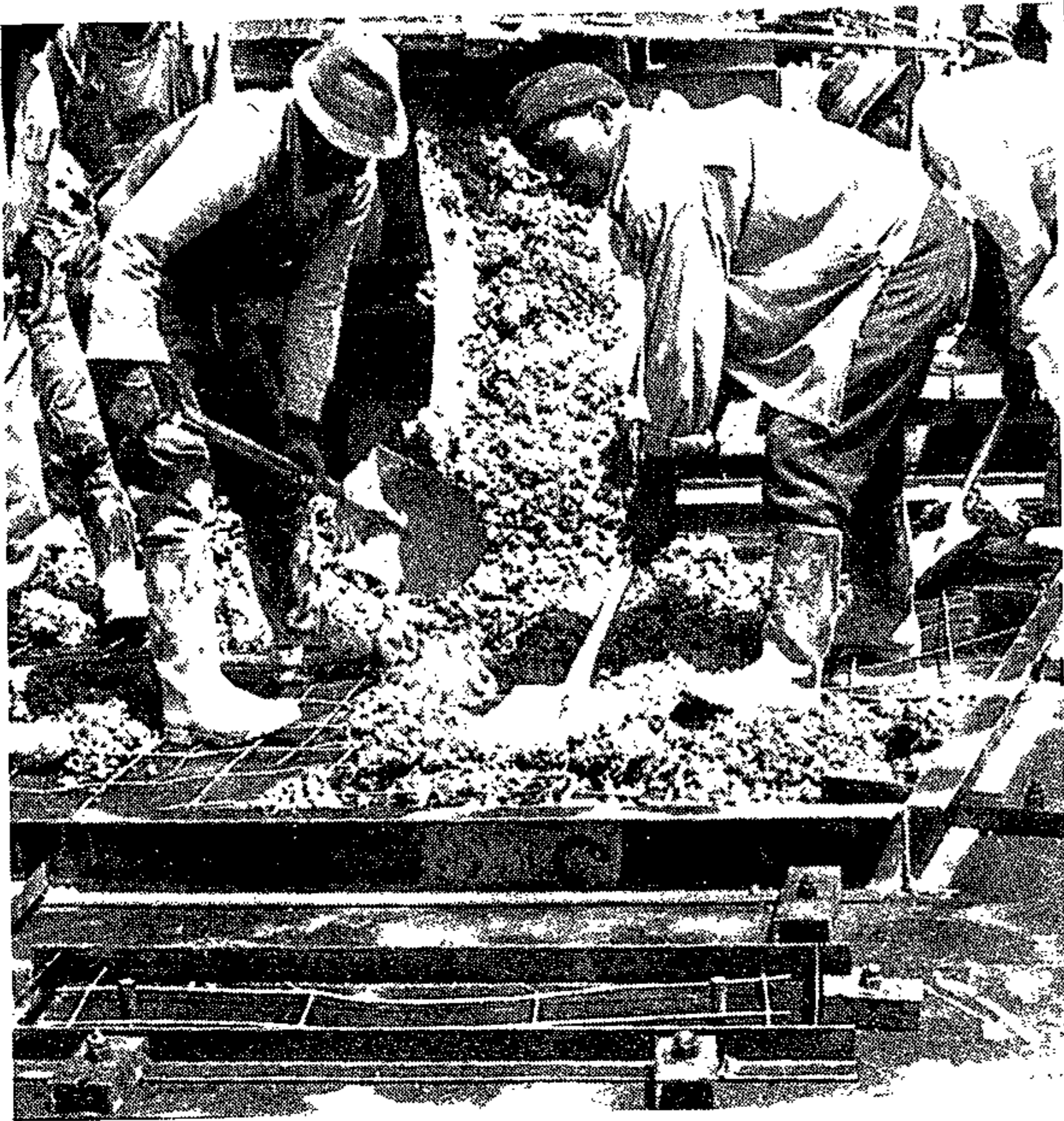
Construction workers spread poured concrete into a mould to cast an element at a precast concrete factory in Umtata. The booming building industry provides much job opportunity for Transkeians.
