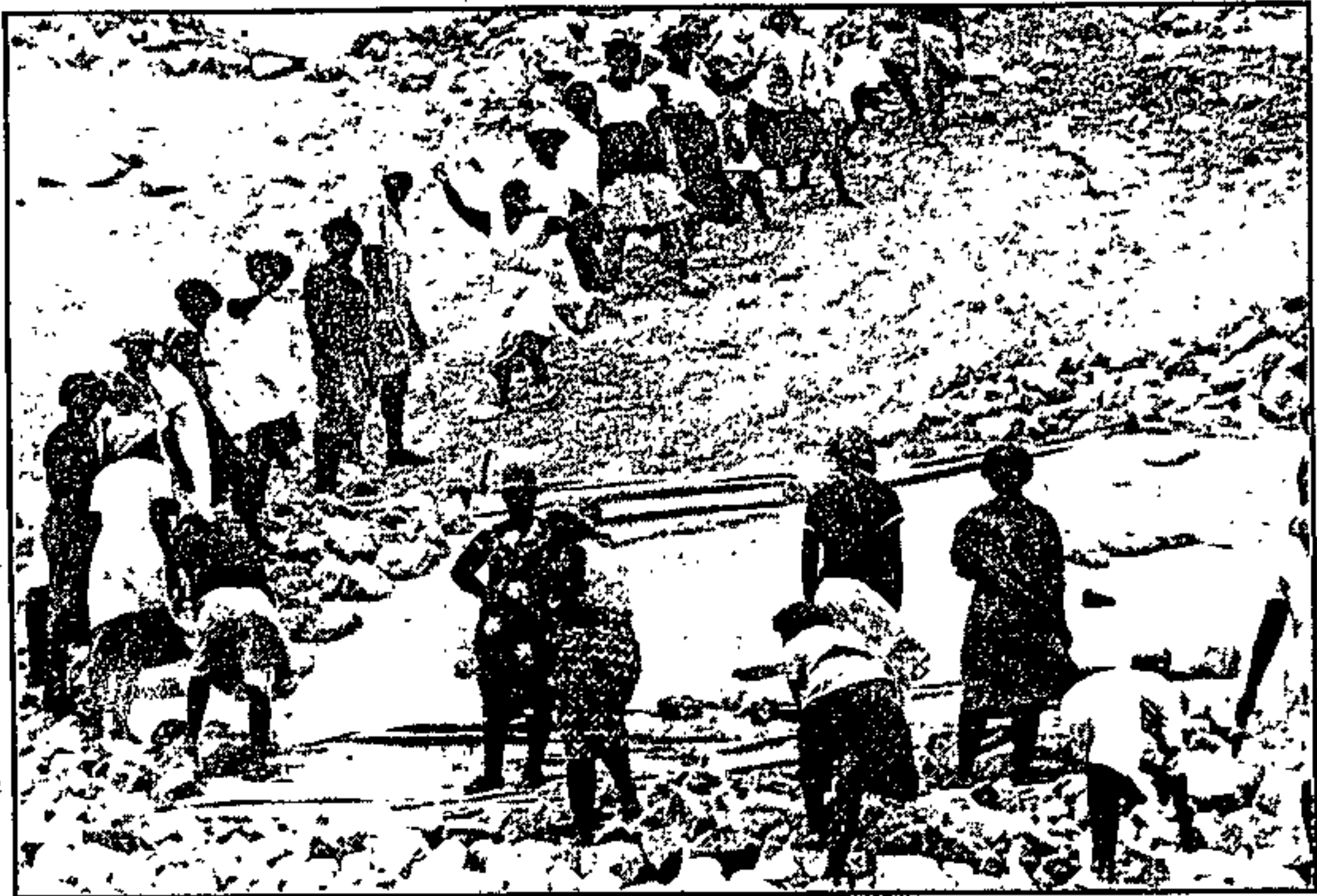
Workers employed at R7 a day lay stones on the outer wall of the collapsed R37 million dam in preparation for repairs. PICS: LEN KHUMALO
