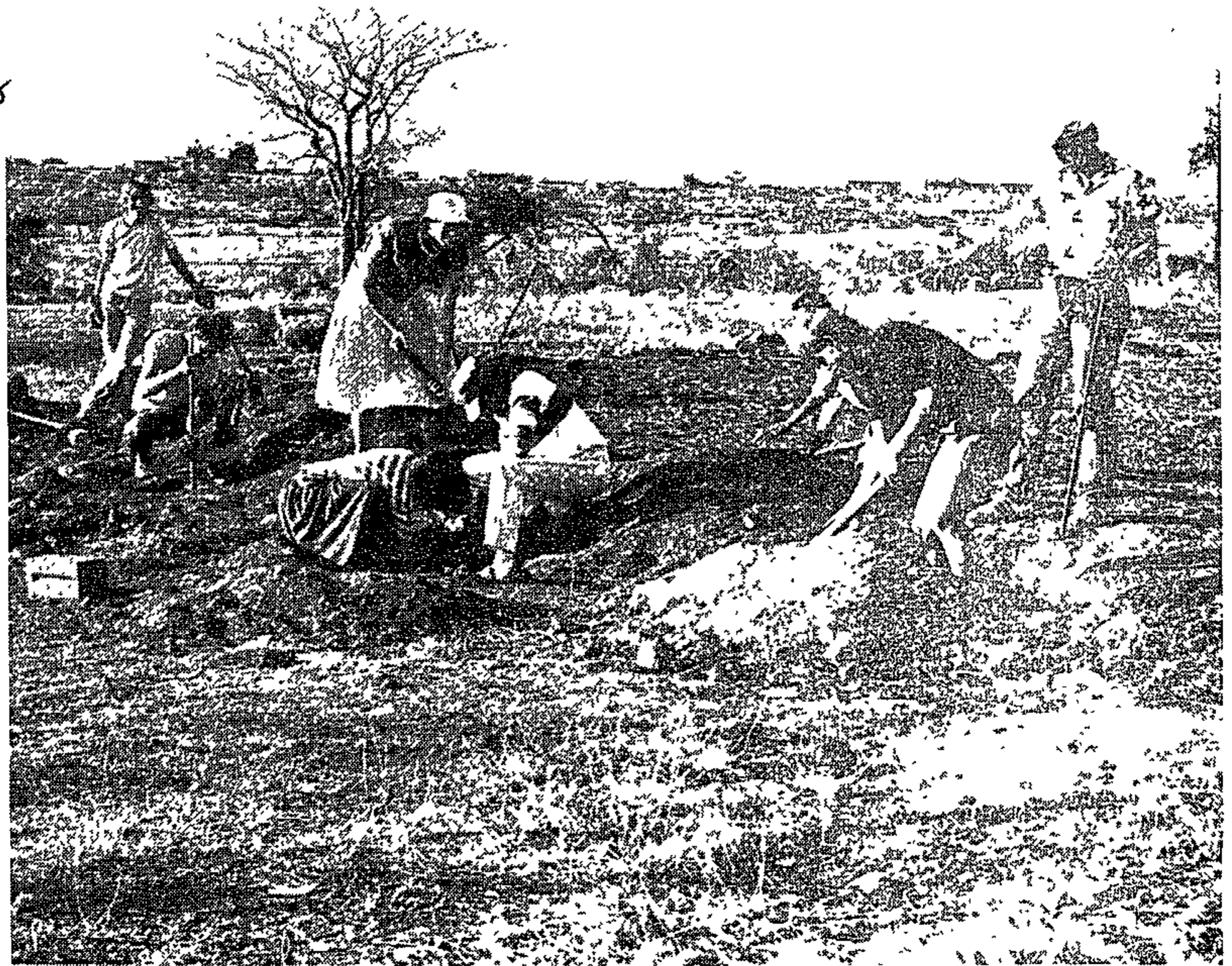
Pretoria university students dig foundations for a church at the Phalalani refugee camp in Gazankulu.
