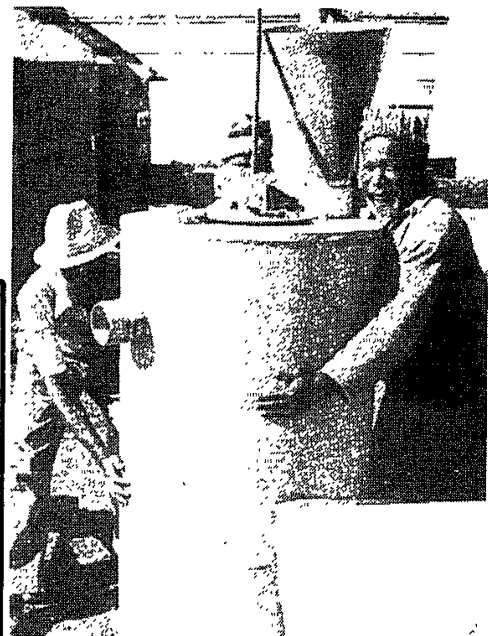
A biogas toilet unit being installed at Jamesdale.
