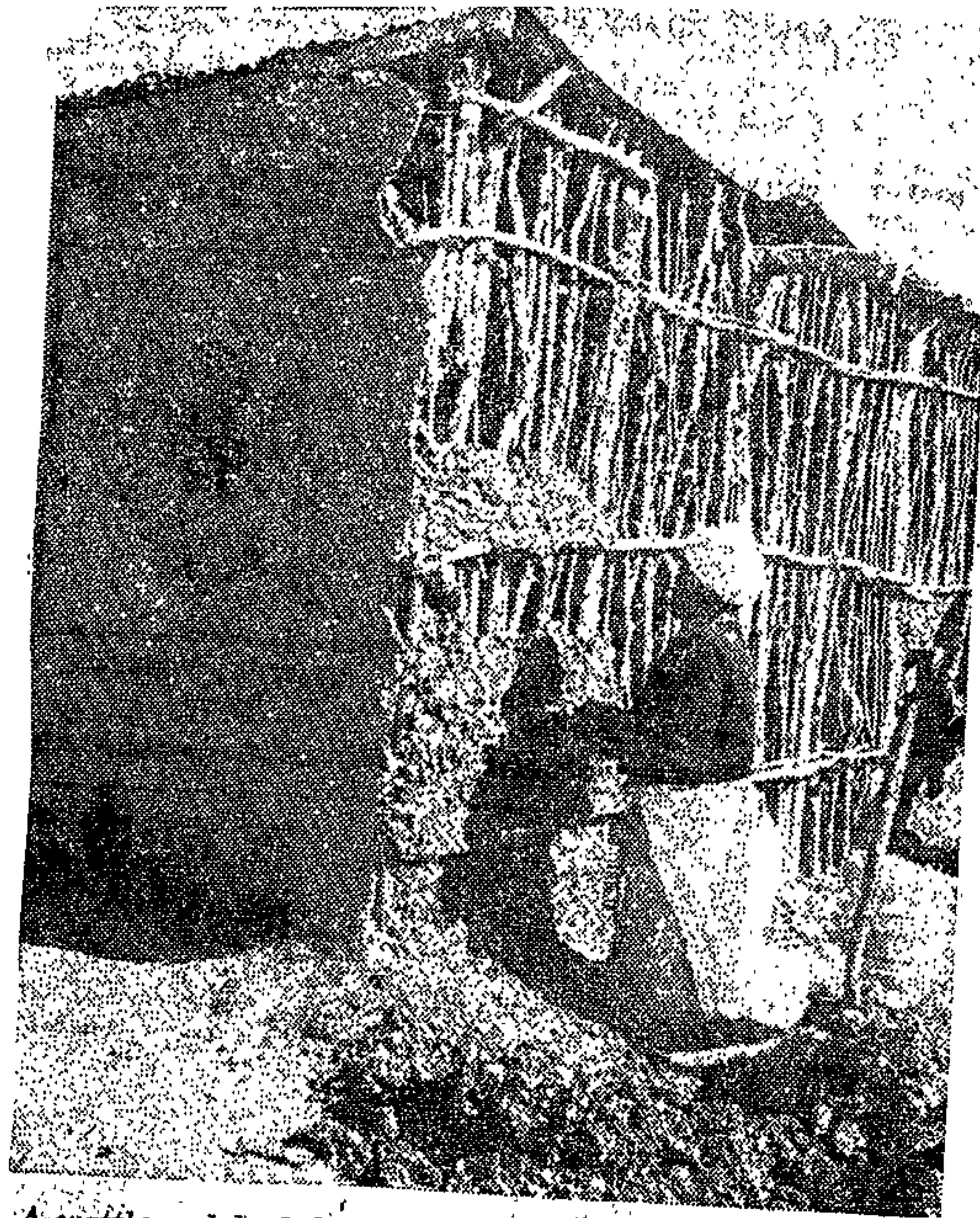
A wattle-and-daub home under construction at Heaton Trust Farm.
