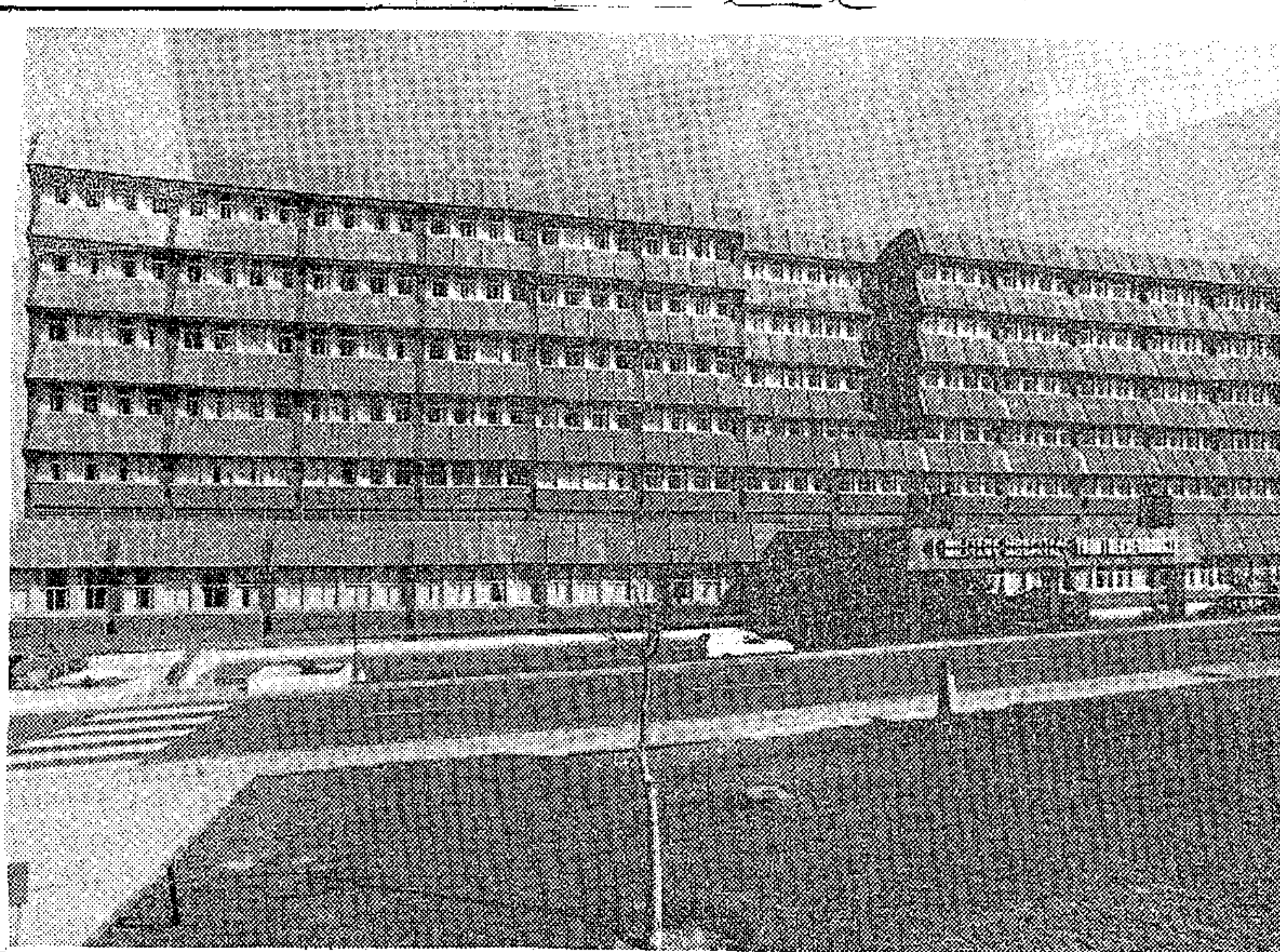
The new 1 Military Hospital has overhanging panels which provide shade from the sun to increase the efficiency of air-conditioning.
