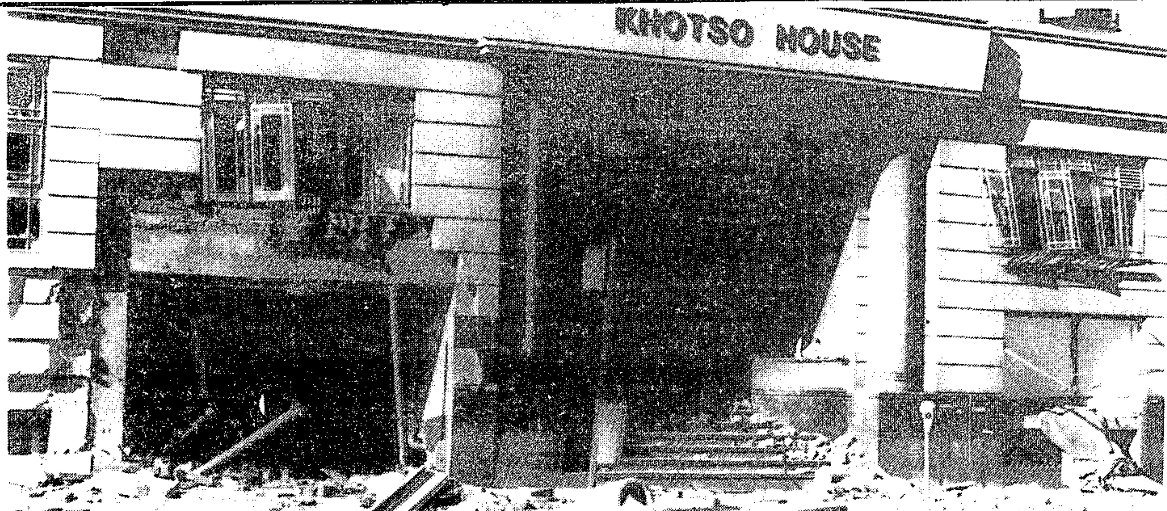
KHOTSO House after it was bombed on Wednesday morning.
