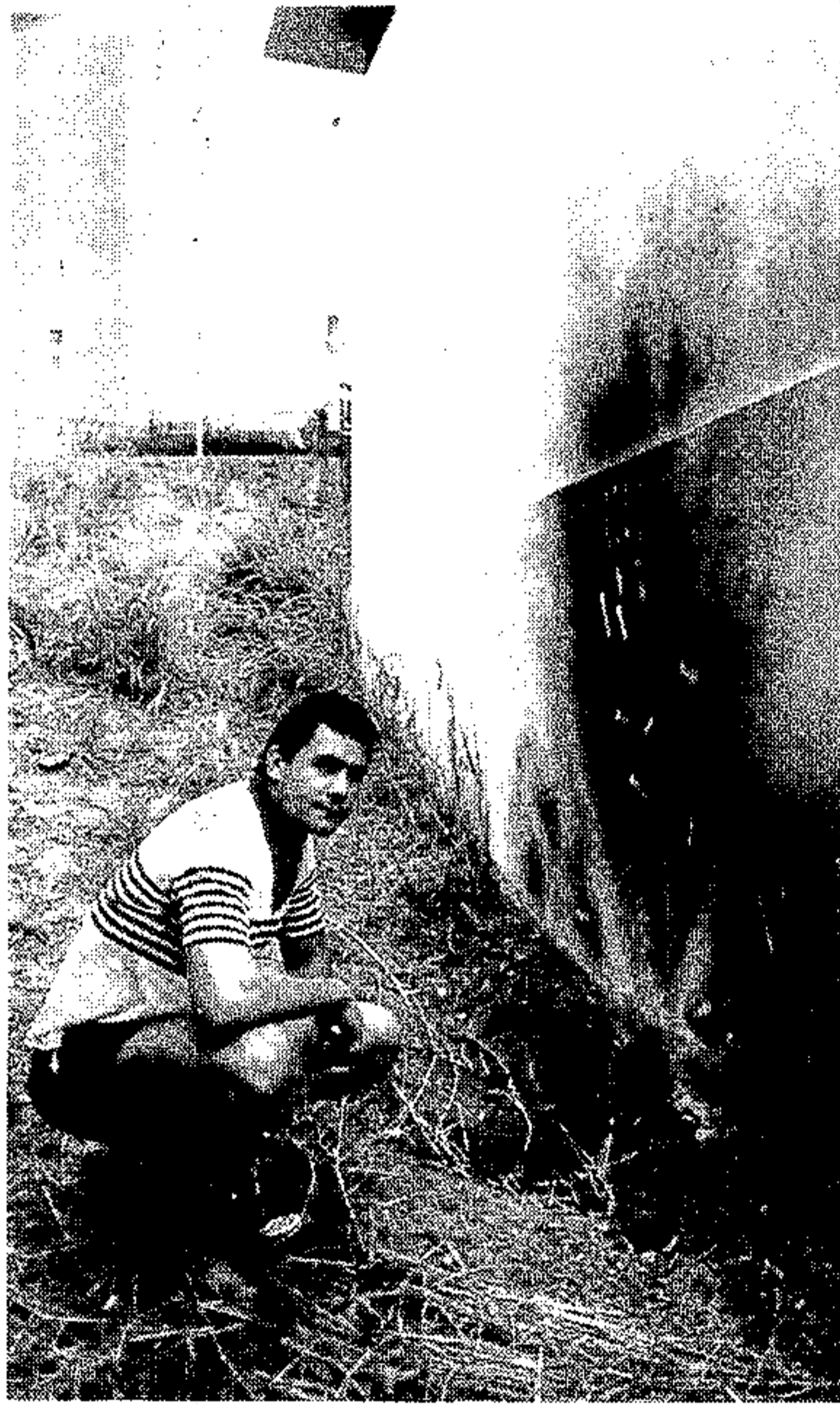
Mr Gary Hoek, who lives across the road from the sub-station, inspects the damage.
