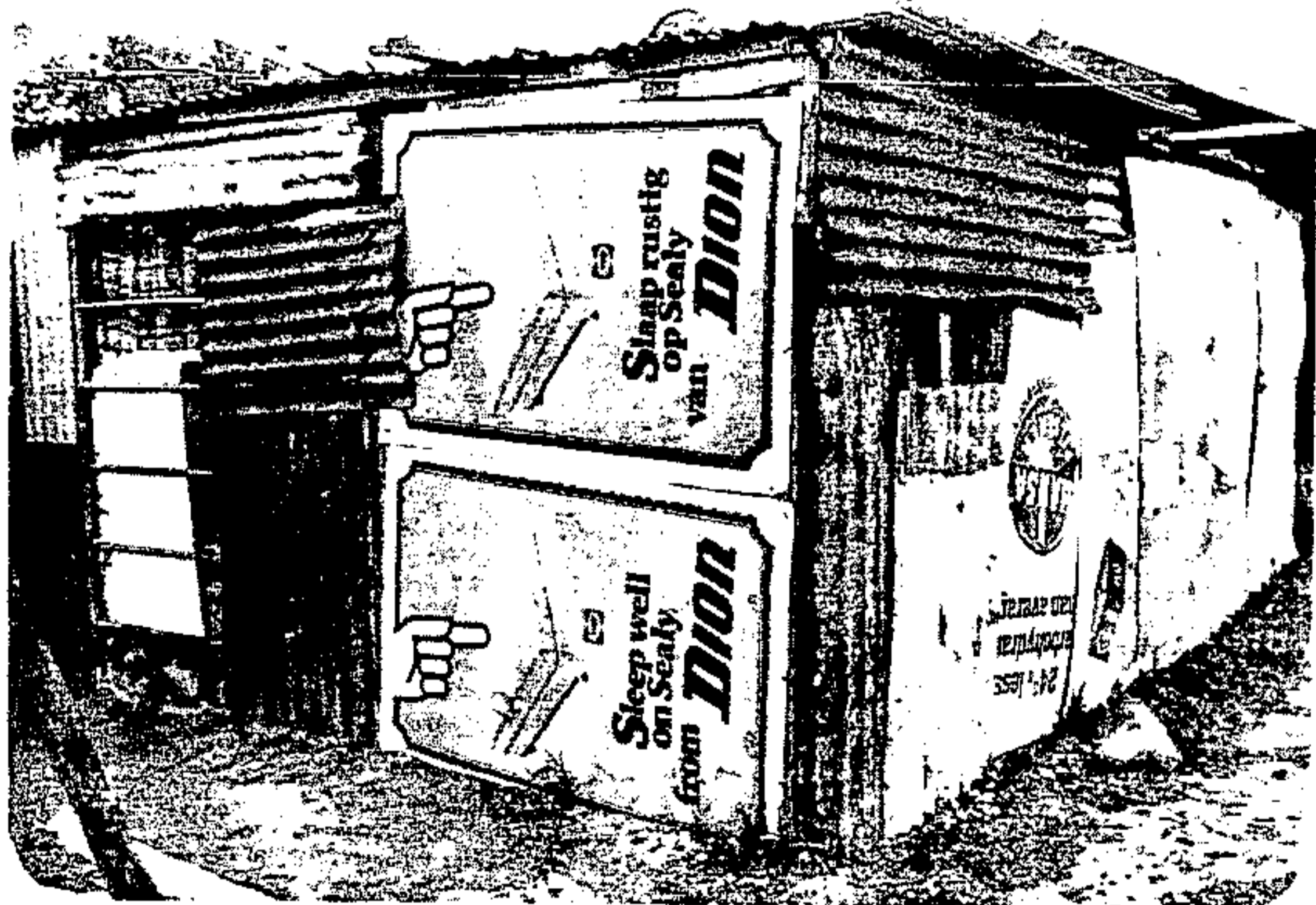
Shacks like this, without even the ironic humour of the hoardings, proliferate throughout SA. The lack of proper service makes them a health hazard. Despite this, the structure has been put together with some skill — there is even a window. Properly encouraged, the owner could no doubt build a house that, besides meeting basic standards of health safety, would be a far more comfortable habitation and a source of pride.
