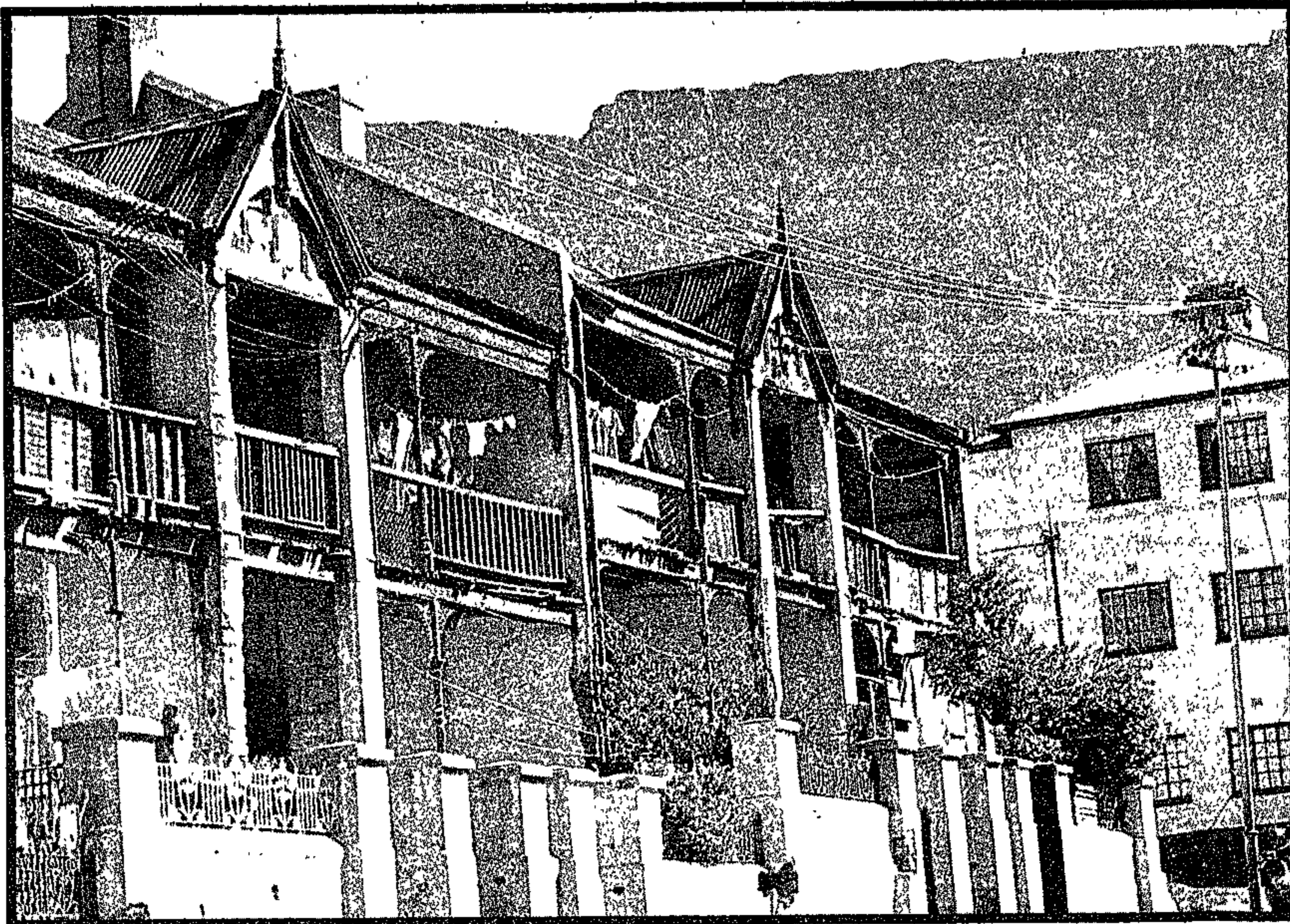
Run down and dilapidated, soon-to-go examples of Georgian Cape houses.
