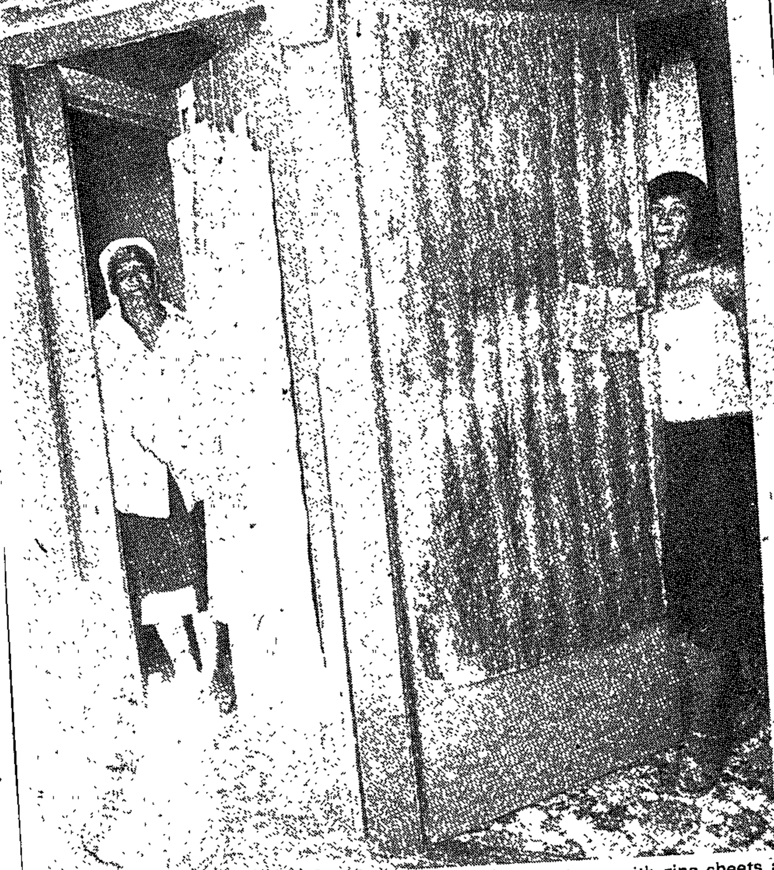
These two Lotus River neighbours covered their smashed doors with zinc sheets after the Divisional Council refused to repair them. Now the families have moved out, but are still paying rent for premises they do not live in. It was the second time the doors had been broken down and the families terrorized.
