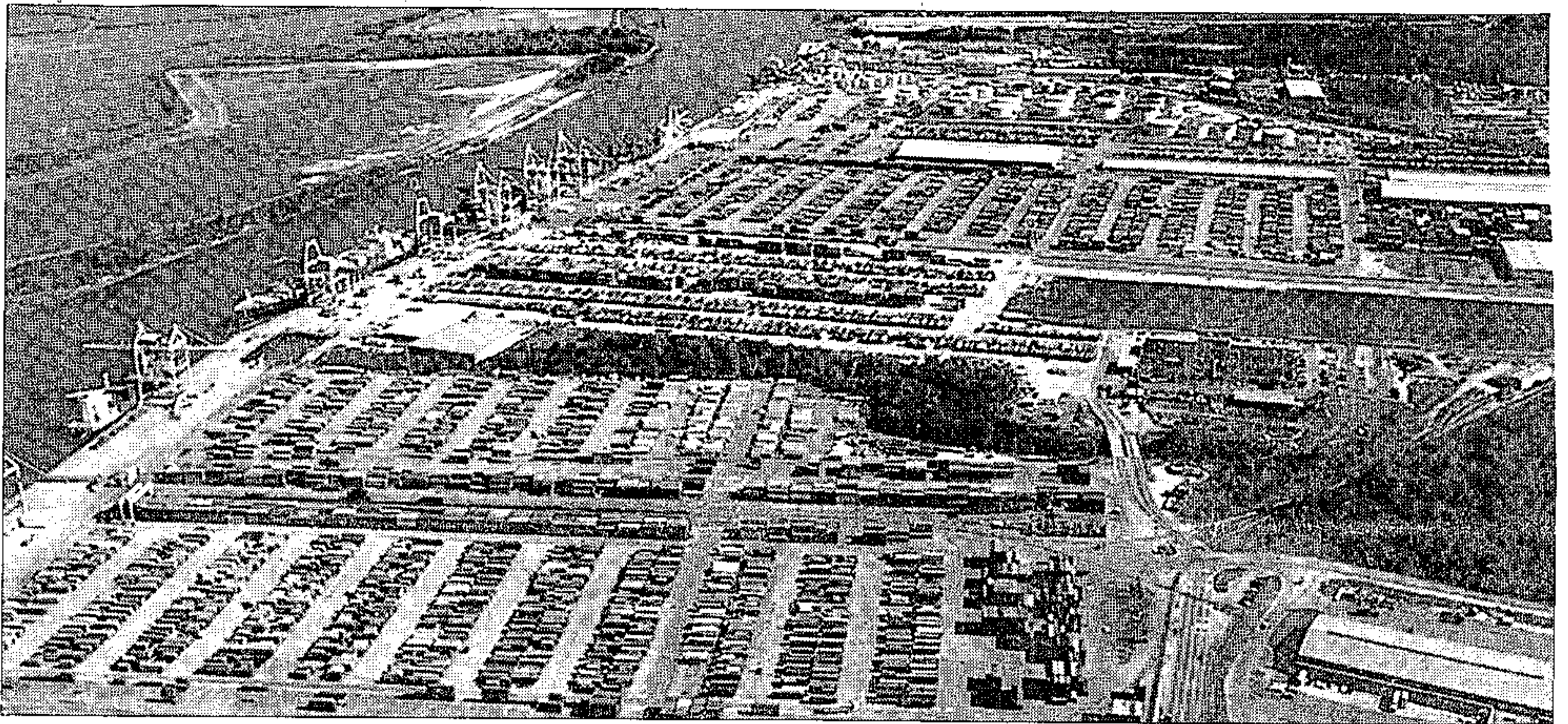
EXPANSIVE GROWTH The port of Savannah in Georgia handles 14 million tons of cargo a year. Its Garden City terminal, shown here, covers 339,27ha. A new container berth covering 59,51ha is under construction
