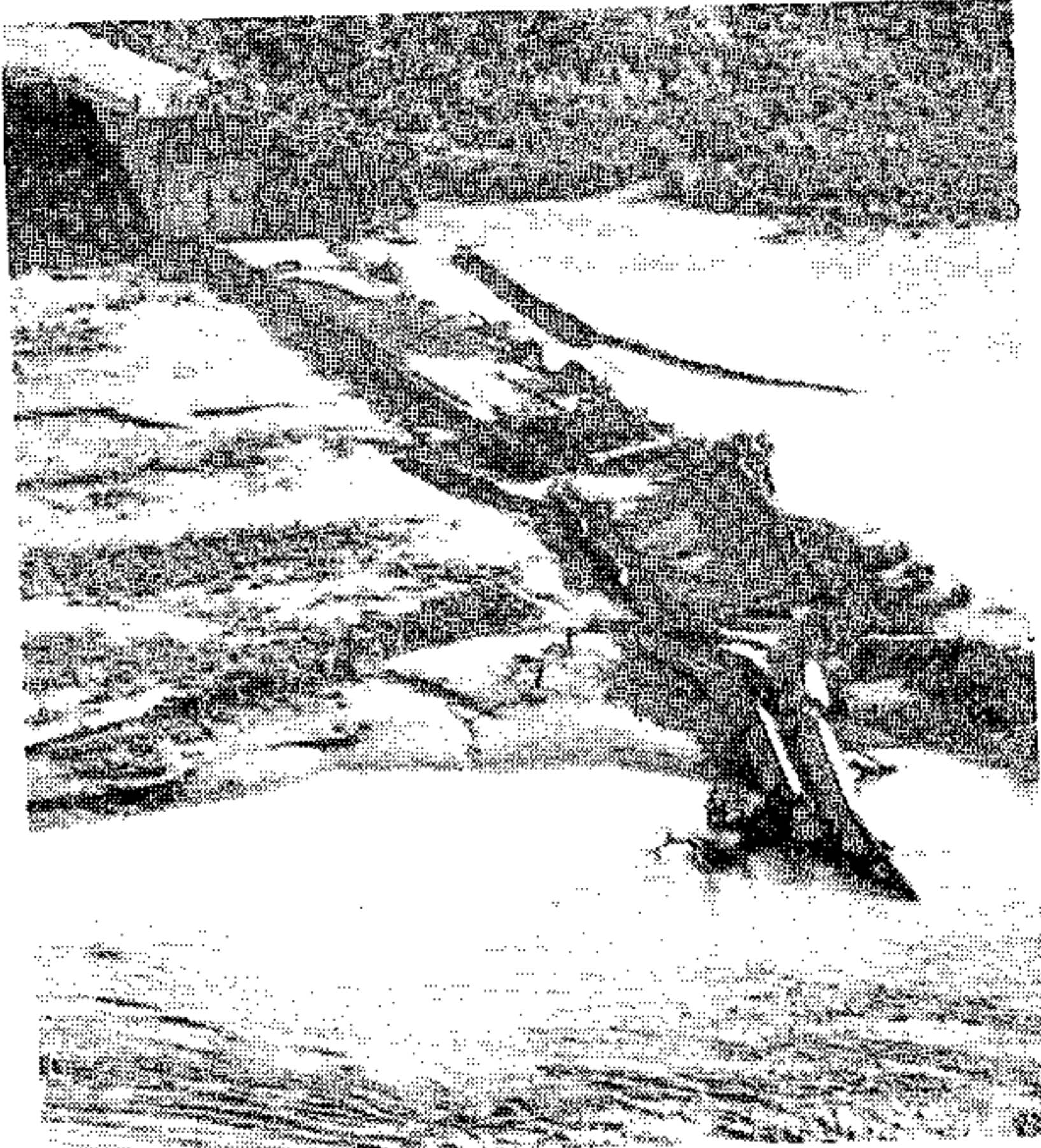
REMAINS ... The fragmented remains of the massive John Ross Bridge over the Tugela River at Mandini which collapsed on Monday night.
