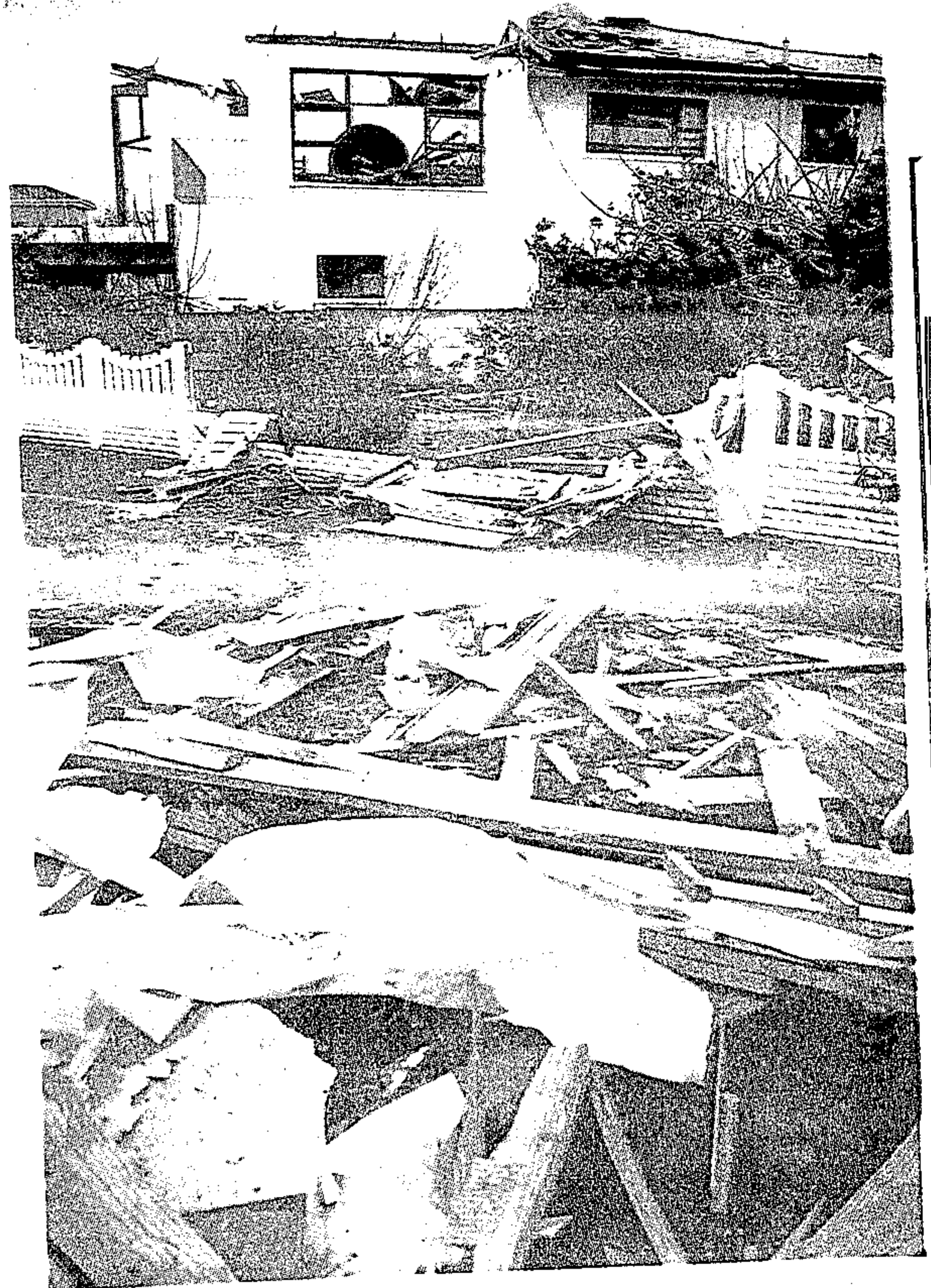
SMASHED: Adela Abduraouf and her family were in their Wetton Road, Wetton, home when the roof blew off and landed half across the road. No one was hurt, but damage was considerable.
