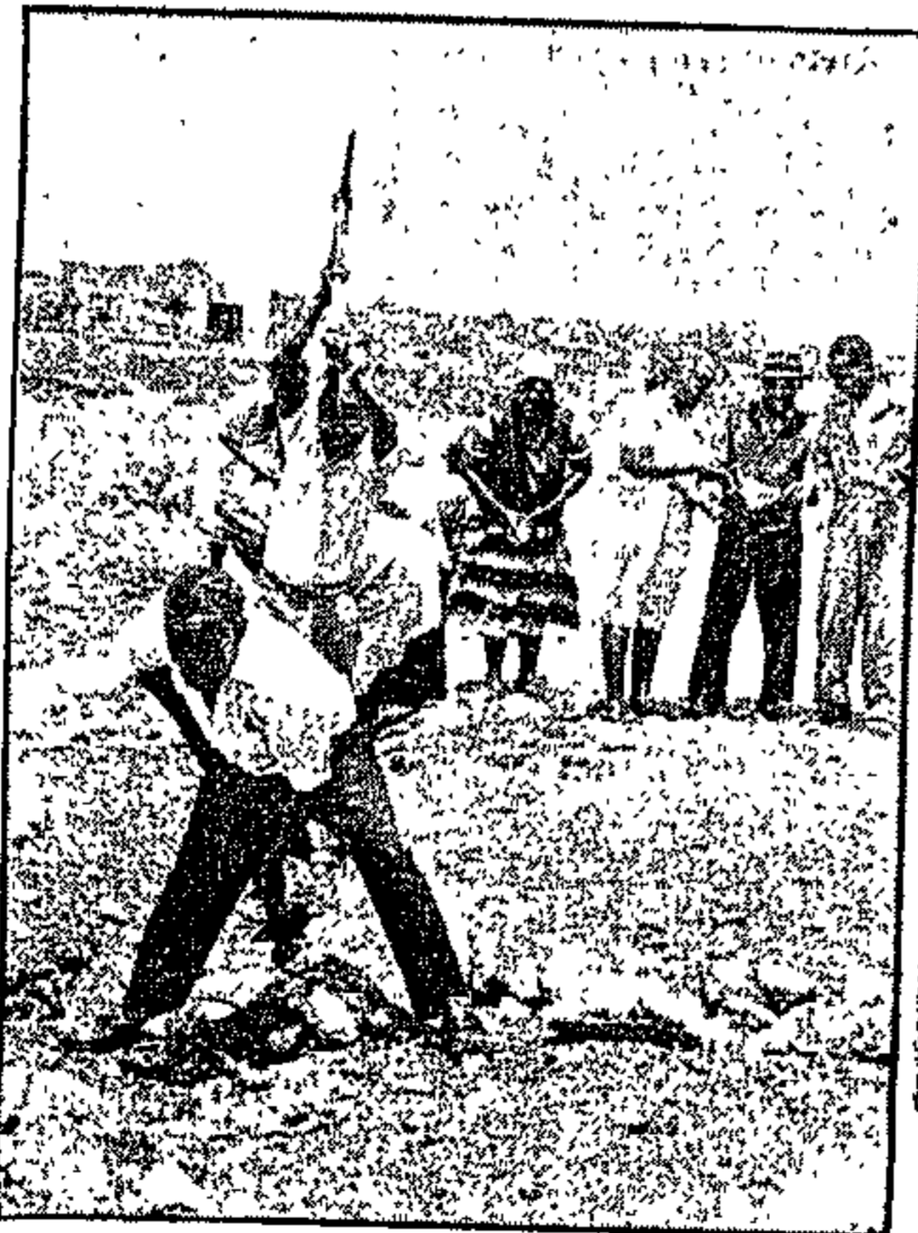
In the trenches... Tooseng Water Committee members show the form which brought water within reach of every resident.
