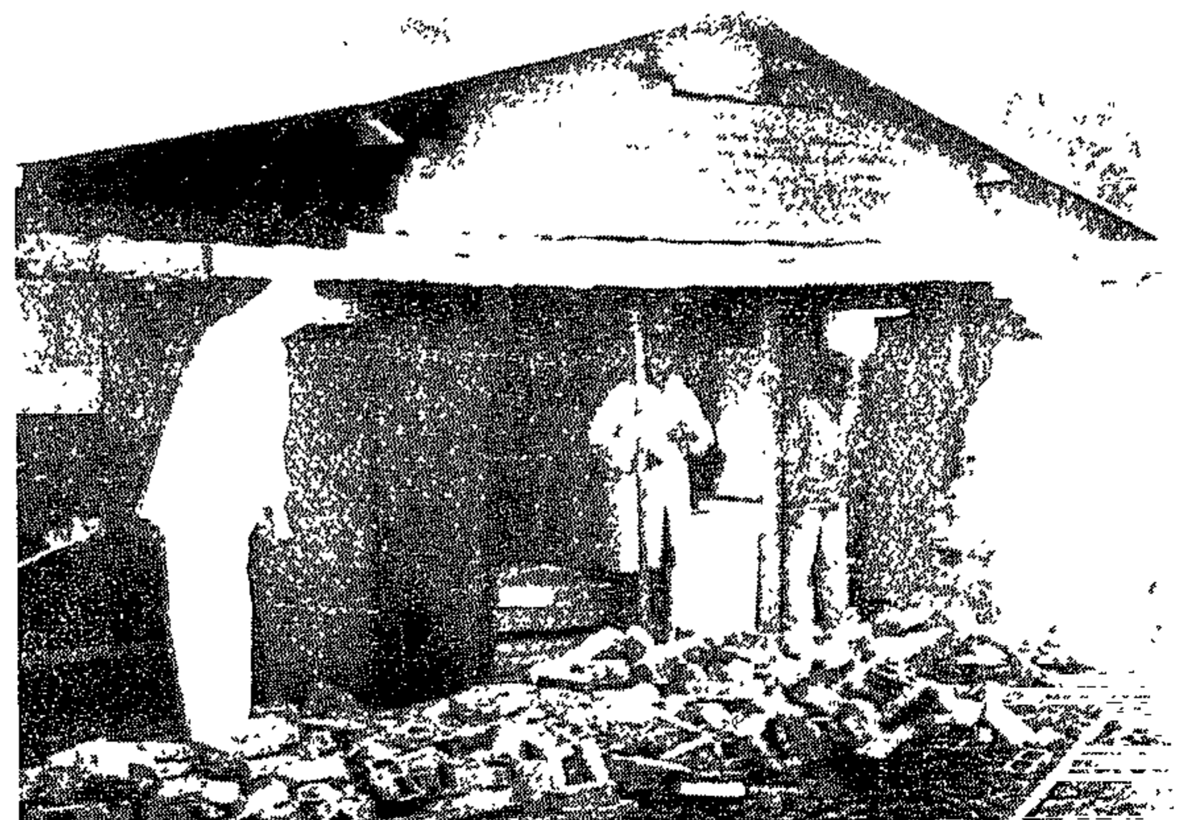
HOMELESS . . . This house in KwaMashu near Durban was destroyed by floodwaters yesterday, leaving a family of eight homeless.
