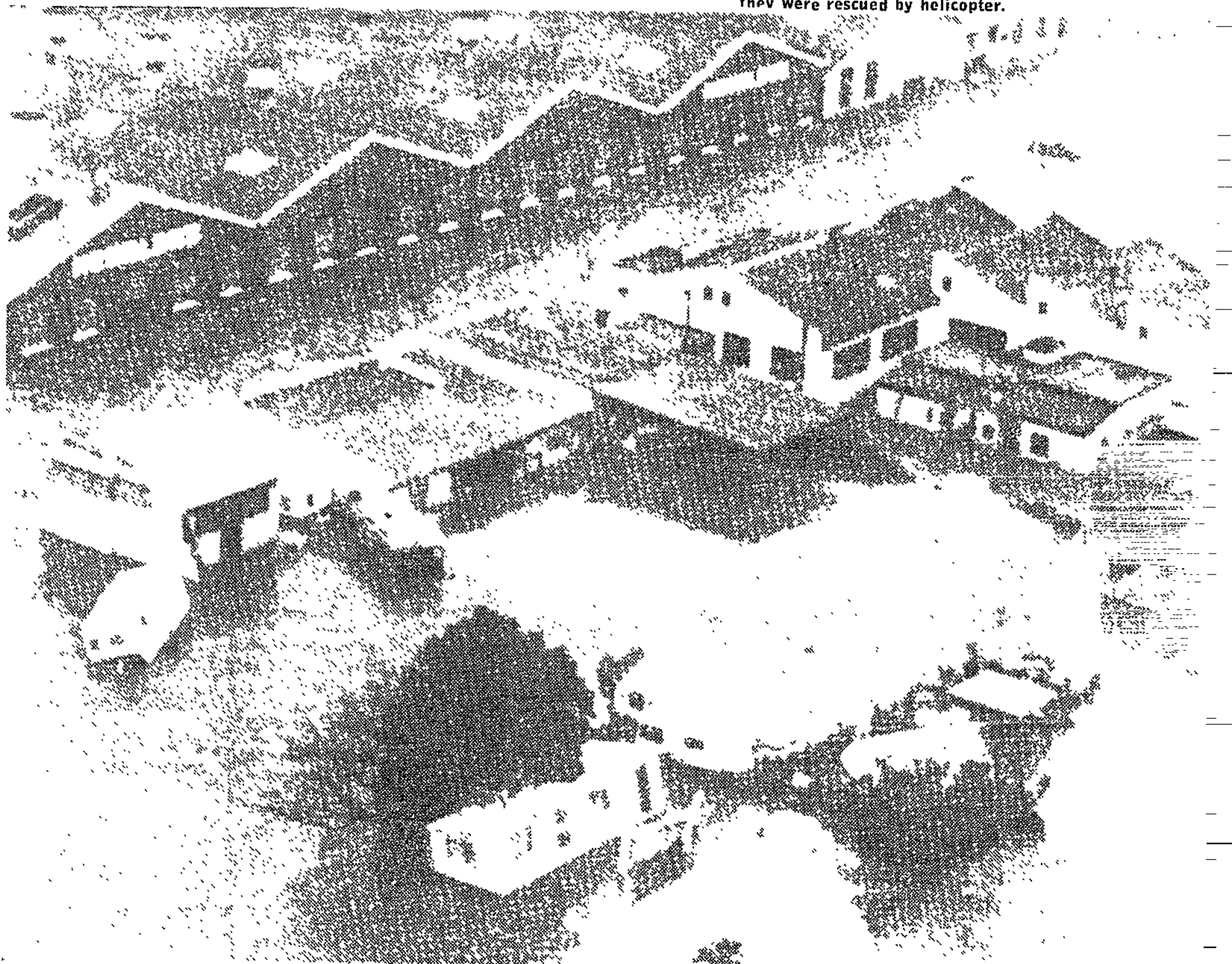
Factory buildings in central Port Elizabeth are threatened by the flood waters from the swollen Baakens River.
