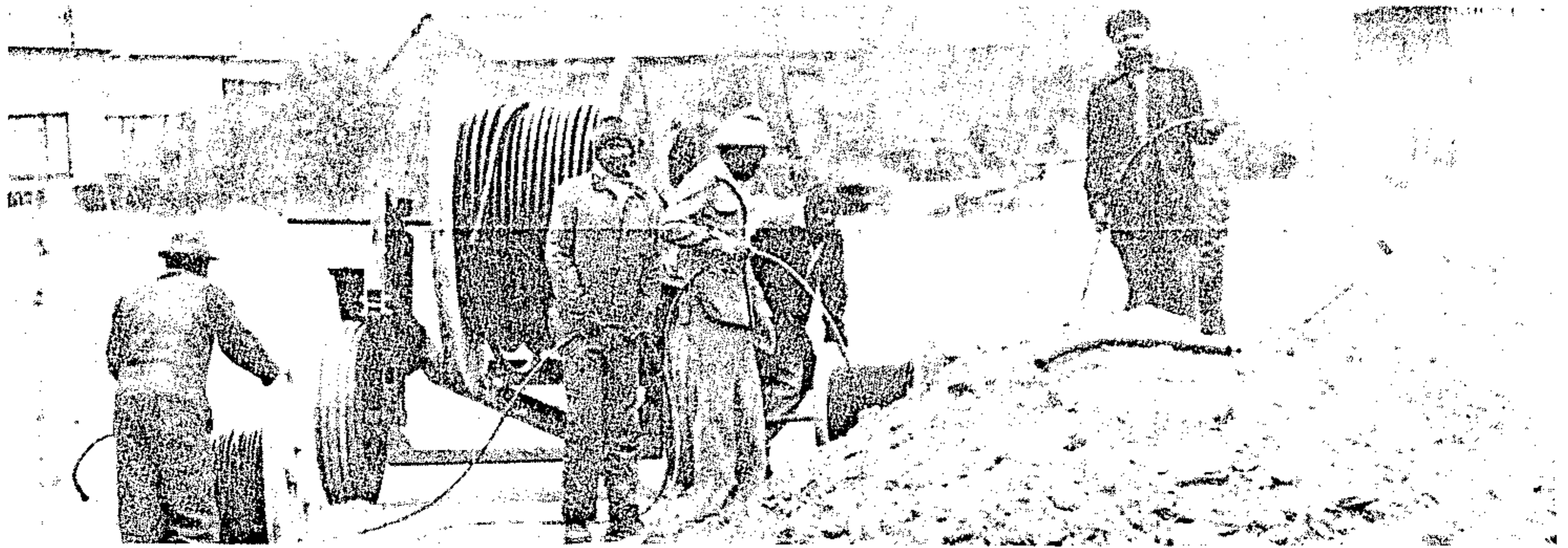
Workmen busy laying cables in one of the major electrification projects in the country. But still there are millions of South Africans who don't have electricity.
