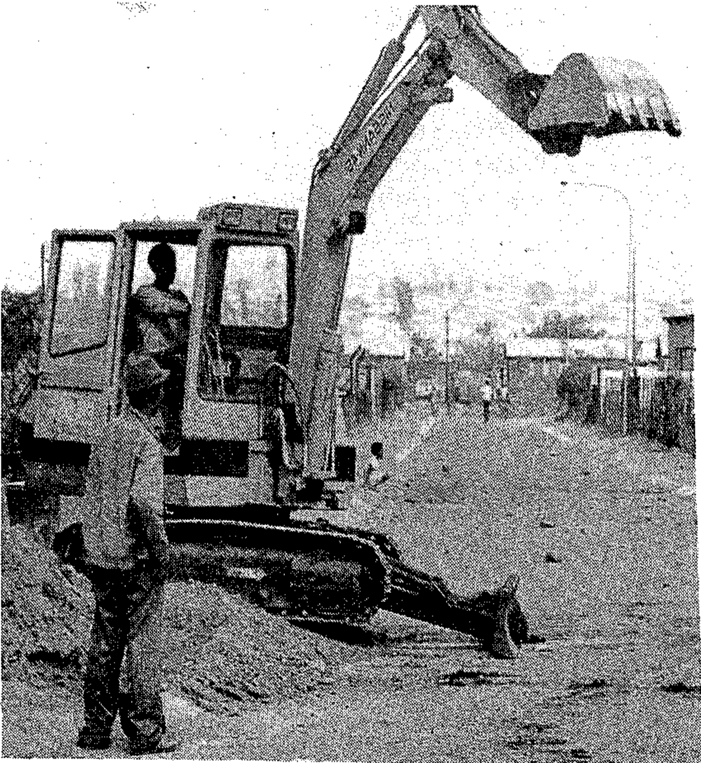
AT WORK: The start of another trench in Meadowlands.
