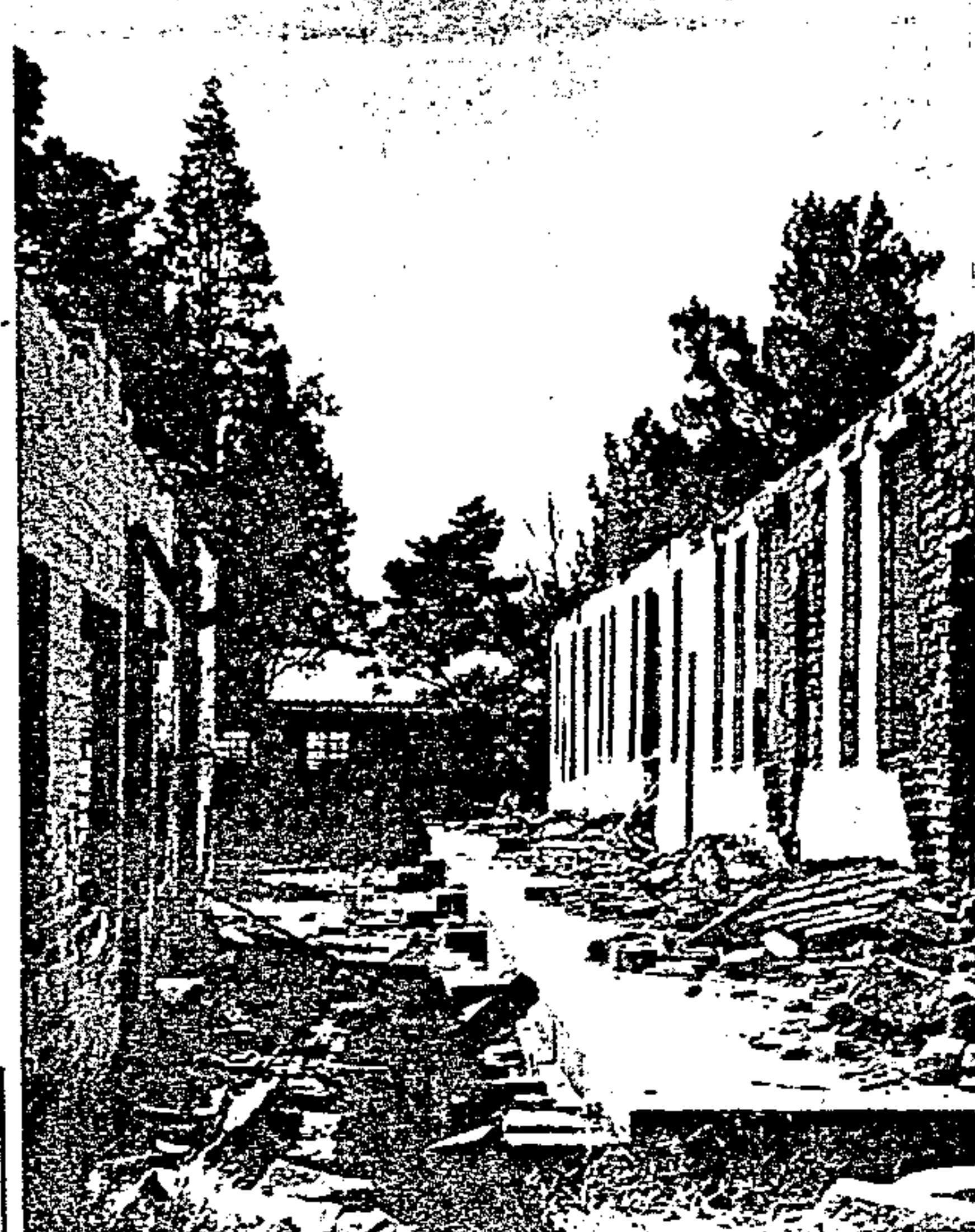
The roof, doors, window-frames and even bricks have been vandalised.
