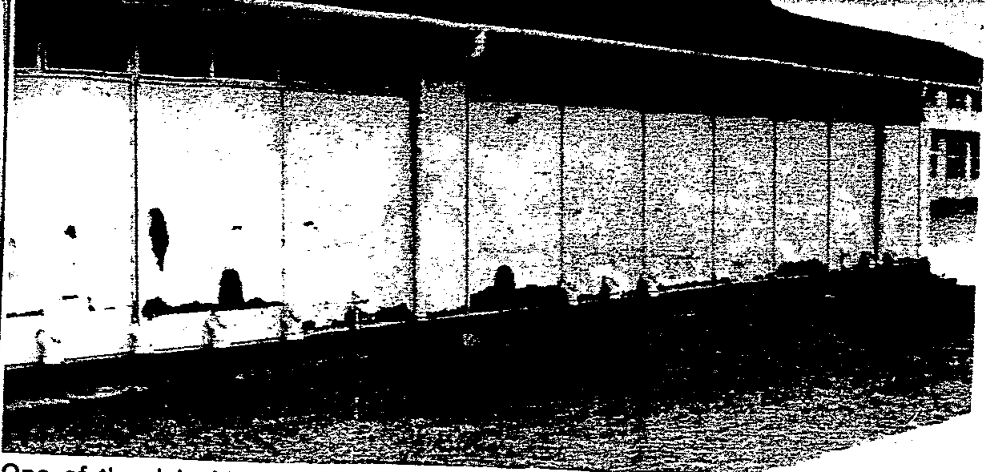
One of the delapidated prefabricated classrooms at the Fairvale High School in Wentworth.
