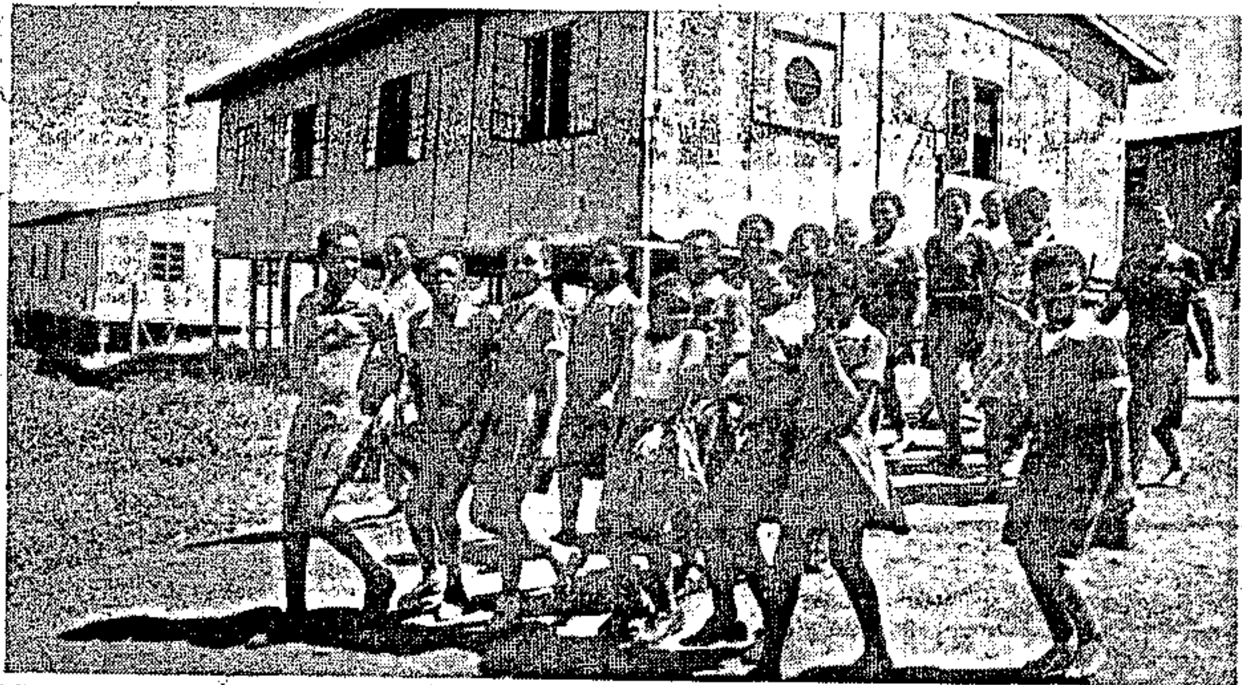
Time and the weather have taken a cruel toll on Patensie's Masisebenze Primary School. Teachers fear for the safety of their 200 pupils because of the condition of the wood and hardboard building.
