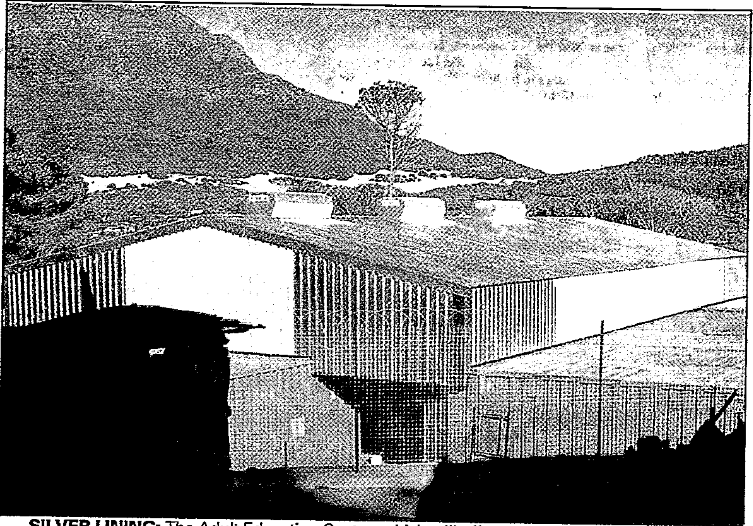
SILVER LINING: The Adult Education Centre, which will offer a variety of opportunities for upliftment at the Imizamo Yethu informal settlement in Hout Bay, is nearing completion.
