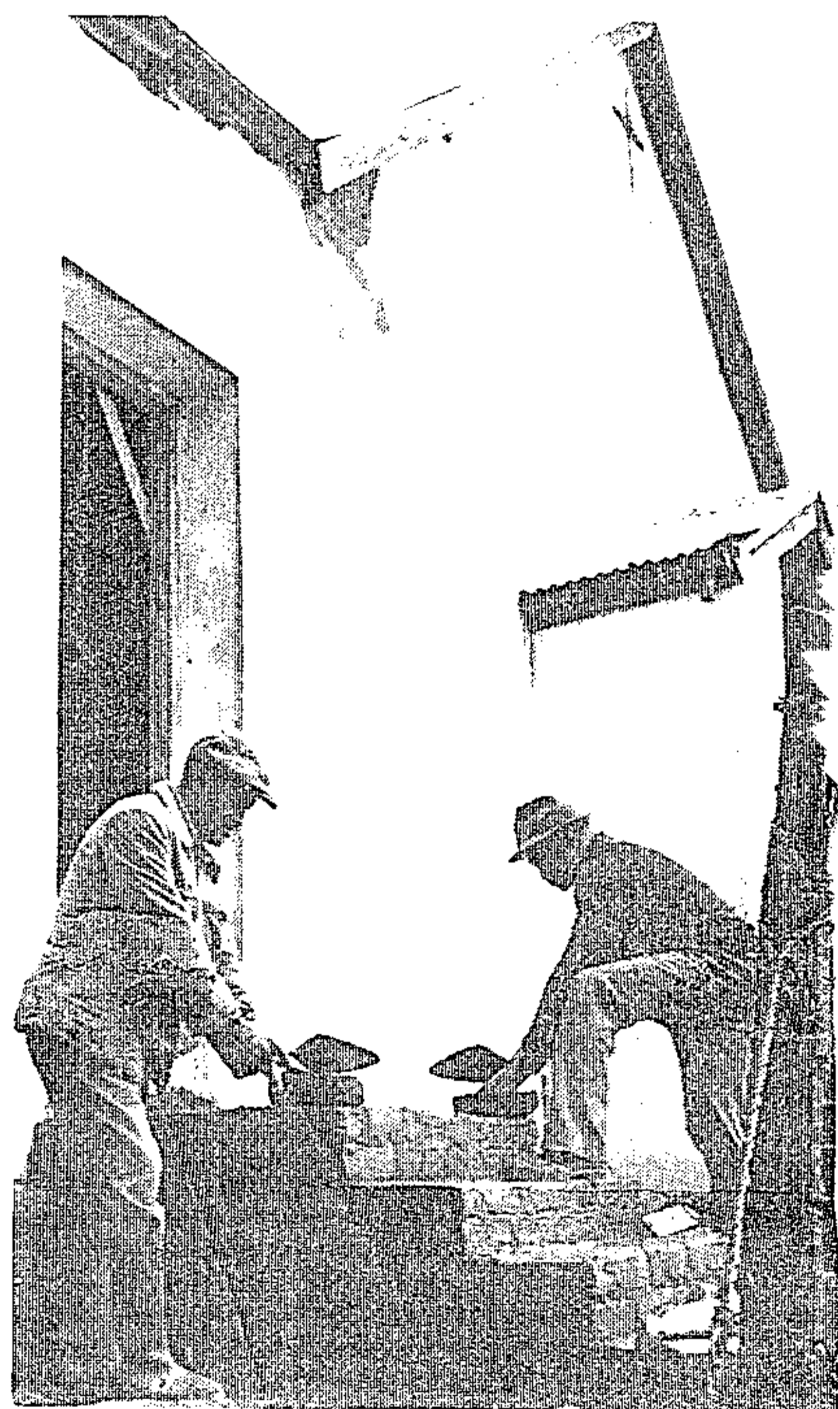
Mr MARTIN APOLLIS and Mr HERMAN MICHAELS helping to convert a disused church into classrooms for coloured secondary pupils in Somerset East.
