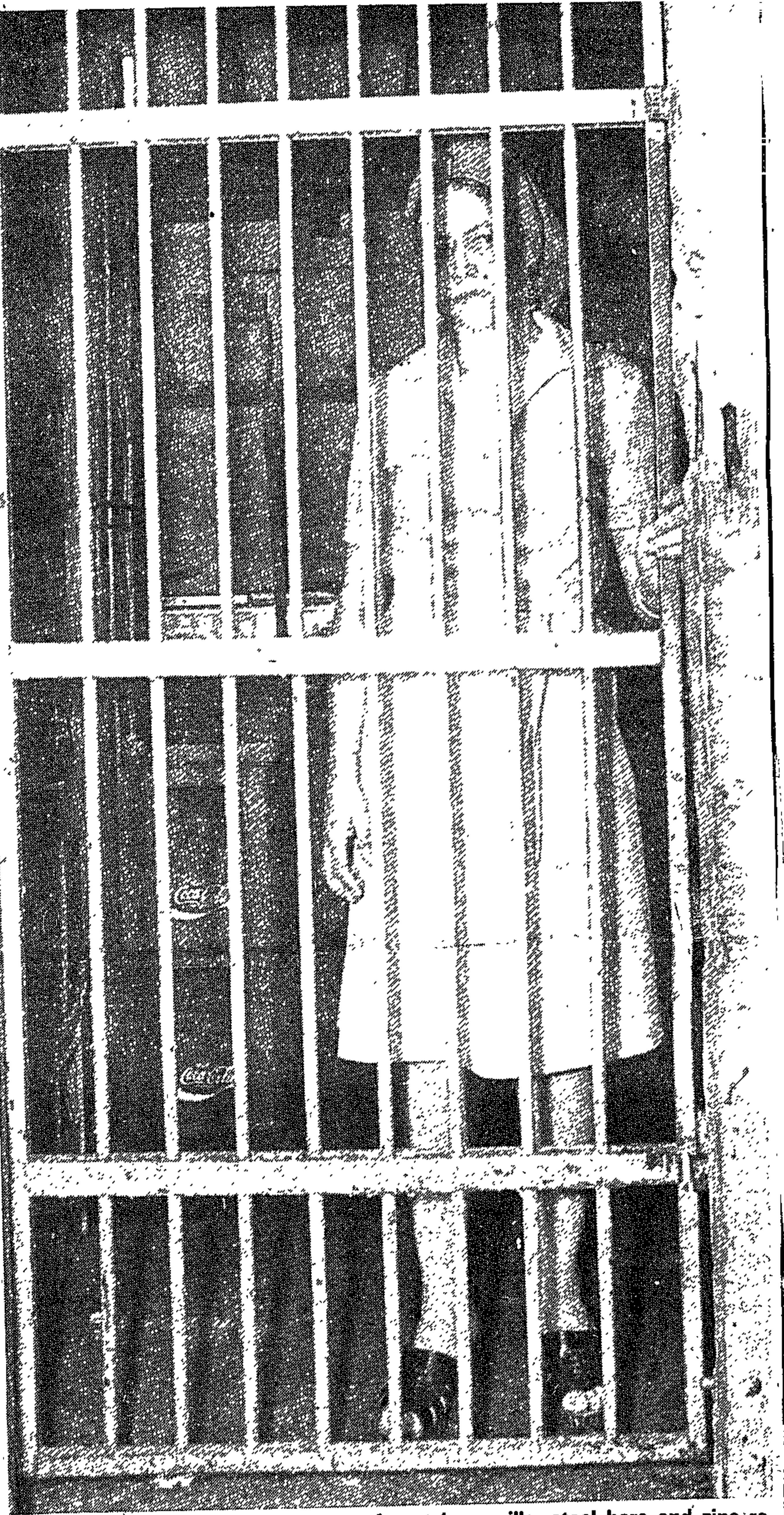
Mrs Abeda Osman in the doorway of cast iron grills, steel bars and zinc-reinforced wooden doors which the burglars hacked their way through.
