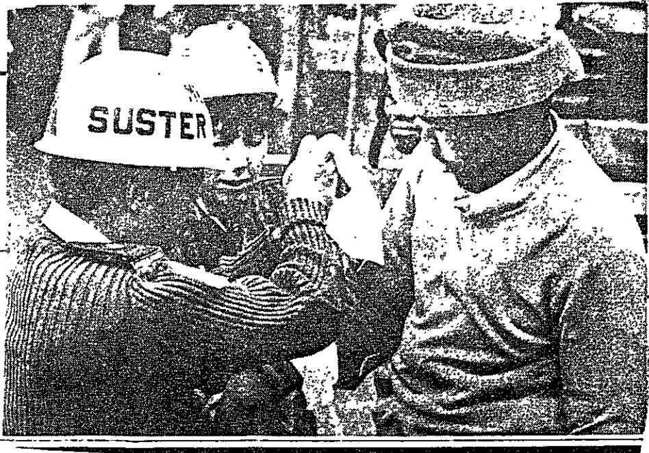
Firemen and Metro workers carry a worker's body from the Hout Street-Burg Street demolition site after a wall collapsed today.
