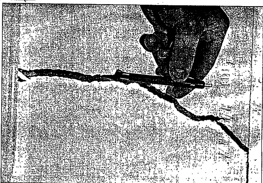
Wall canyon -- shoddy workmanship caused a massive crack in this wall, but in future there will be severe consequences for the builder.
