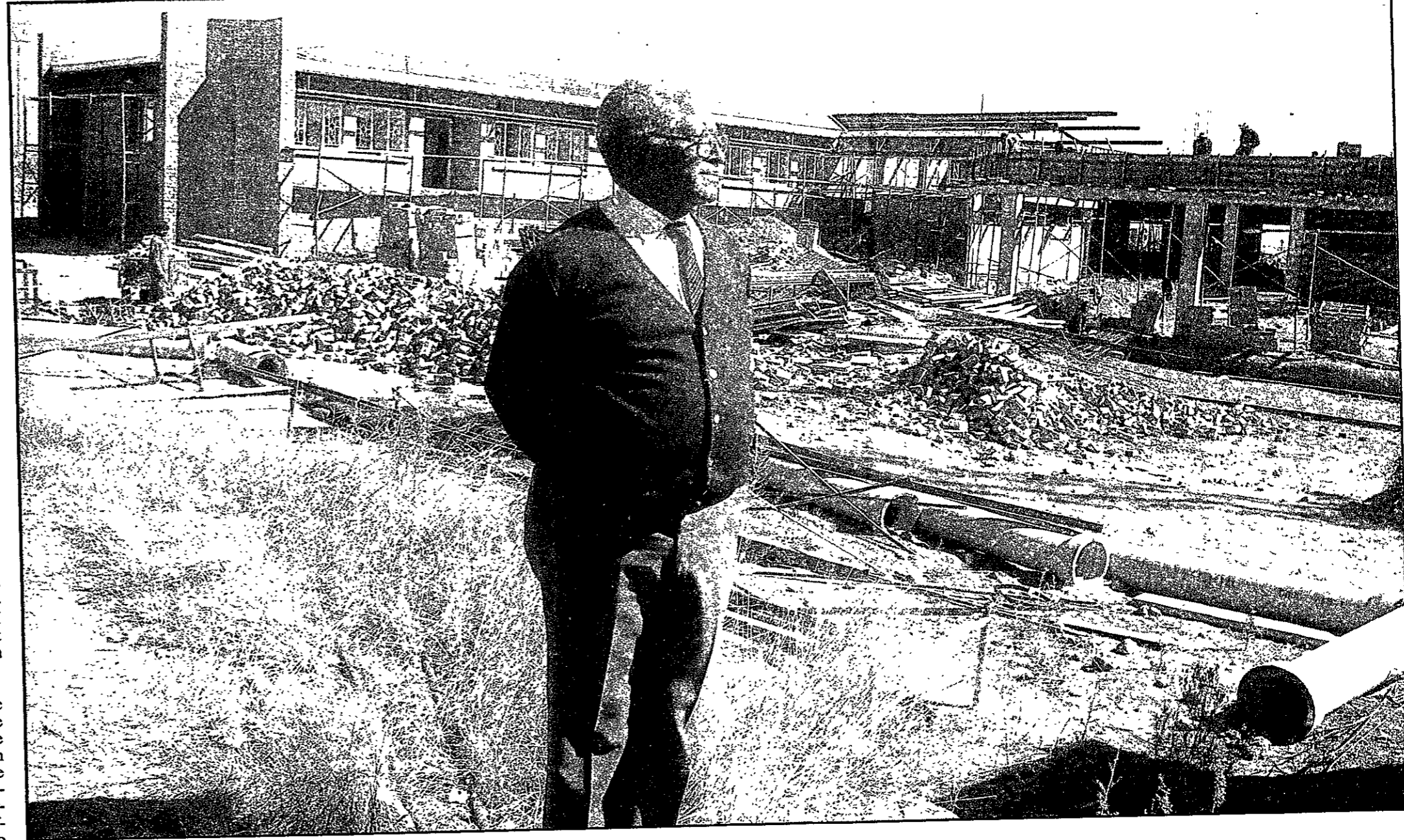
Nafcoc chairman Dr Sam Motsuenyane stands in front of Nafcoc's R5-million leadership centre, which is under construction.
