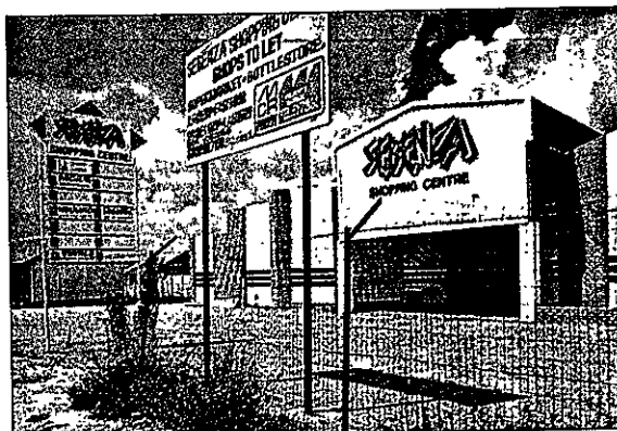
Township shops in Vosloorus ... still a clear field
