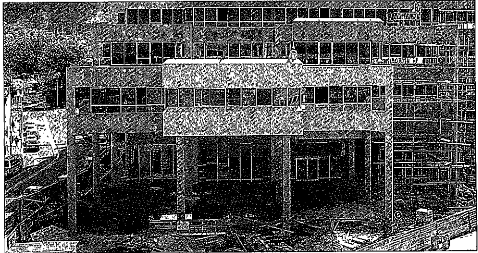
Sanlam's Sanclare project ... nearing completion
