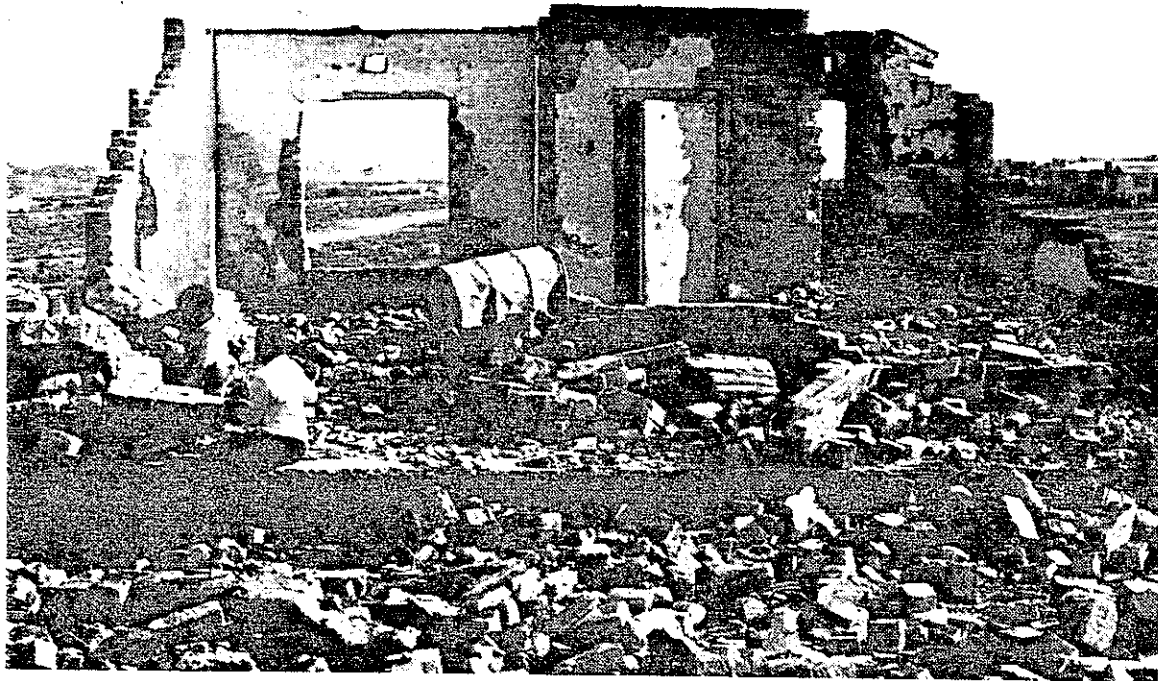
Development board offices in Bongolethu — reduced to a pile of rubble.
