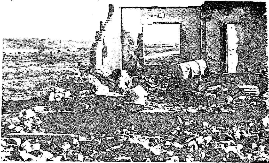
The development board offices in Bongoletu — reduced to a pile of rubble.
