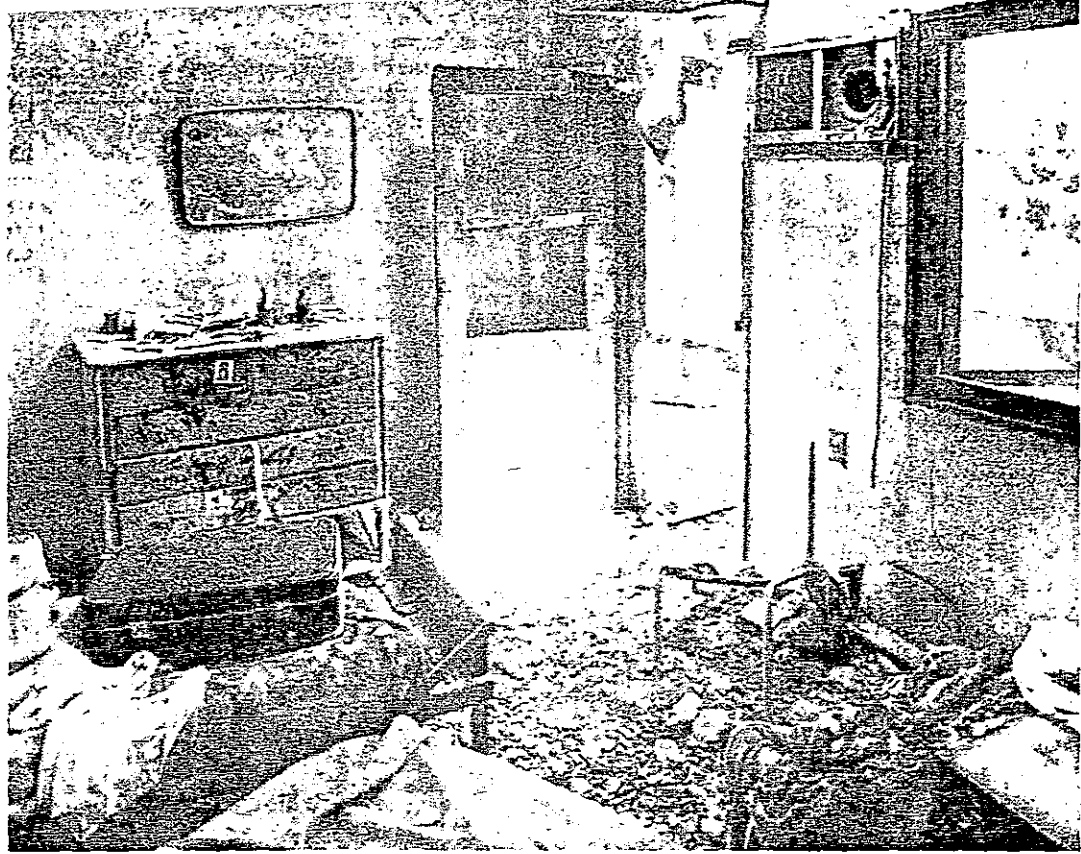
Shattered glass, dust and concrete debris fill one of the rooms at the ANC offices in Maputo which were badly damaged by explosives — thought to have been landmines — planted on the roof.
