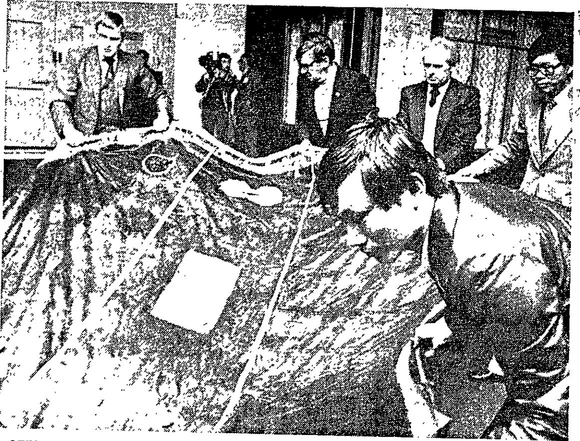
OFFICIALS from the Taiwanese consul general's office and surveyor representatives of the China Corporation Register of Shipping examine the bottom section of the inflatable life-raft from the ill-fated tunny catcher King Chun. The partly inflated rubber raft was found and brought to Cape Town by the Panamanian freighter Victoria 1. Circled in the foreground are two of the numerous patches on the craft.
