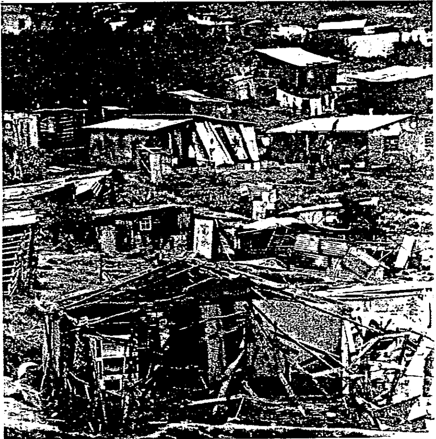
EXPOSED TO THE ELEMENTS: Squatter shacks destroyed in a flood
