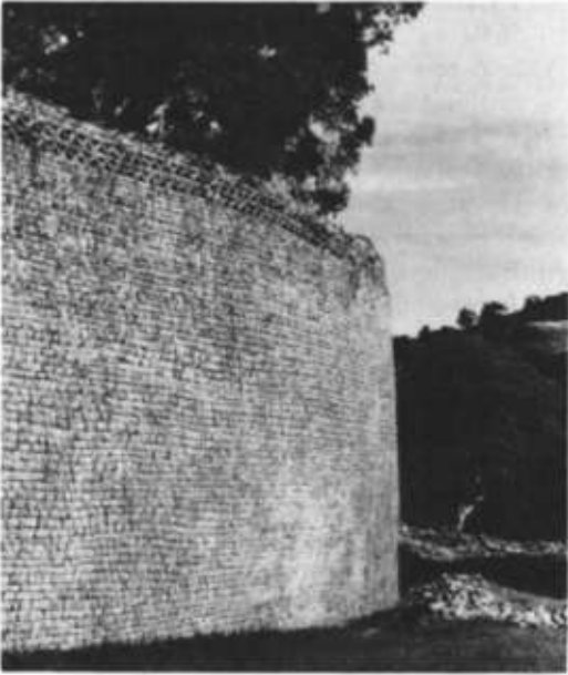
PLATE 21.3 The wall of the Great Enclosure at Great Zimbabwe
