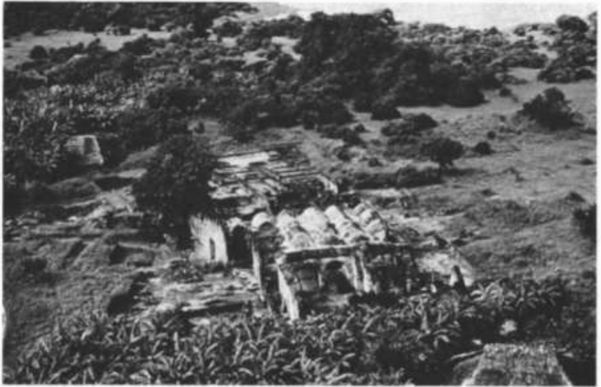
PLATE 18.3 The two adjoining buildings of the Great Mosque at Kilwa
