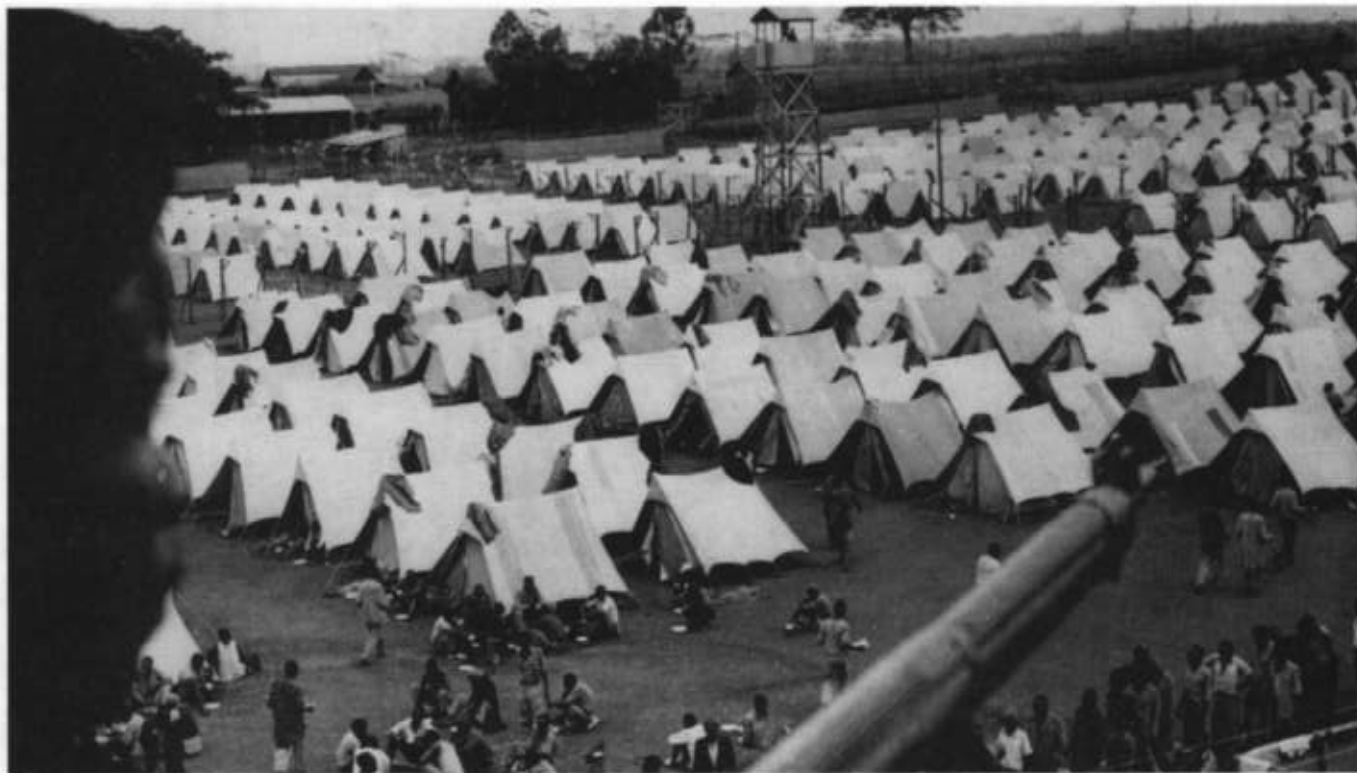
PLATE 9.4 Langata Detention Camp set up by the British during their anti-Mau Mau operations, April 1954
