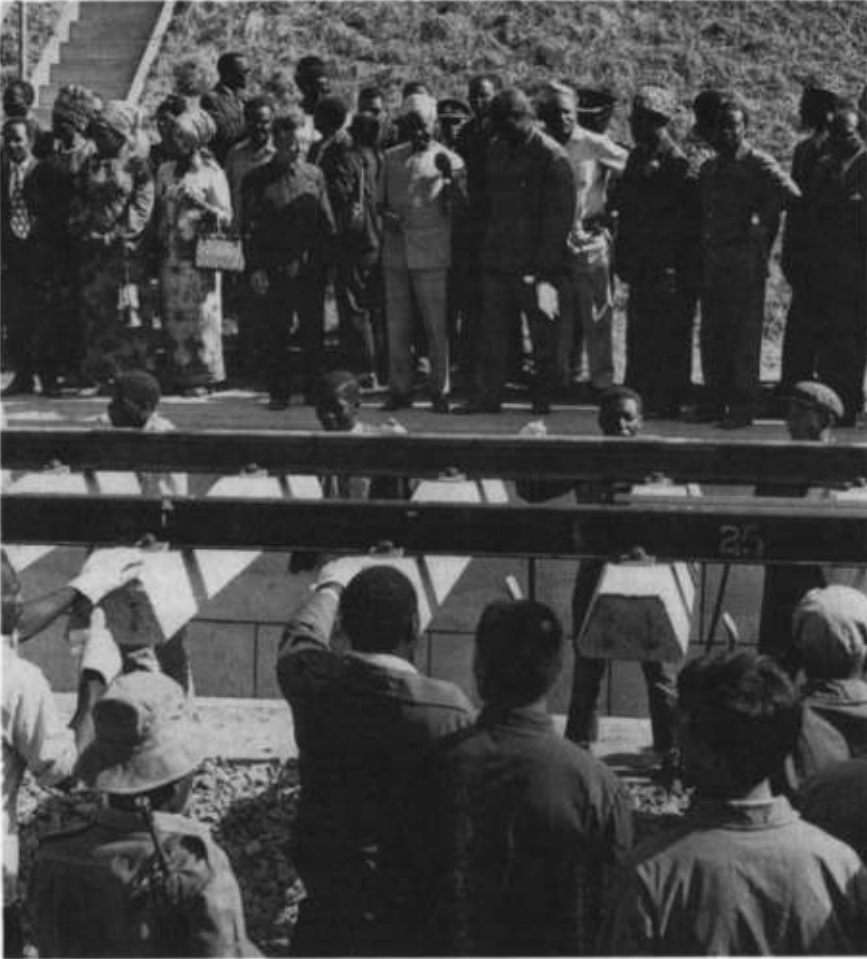
PLATE 27.3 The Chinese-built 'Green Uhuru Railway', Tanzania-Zambia: the laying of the track across the Tanzania-Zambia border, September 1973, in the presence of Chinese officials and Presidents J. Nyerere of Tanzania and K. Kaunda of Zambia
