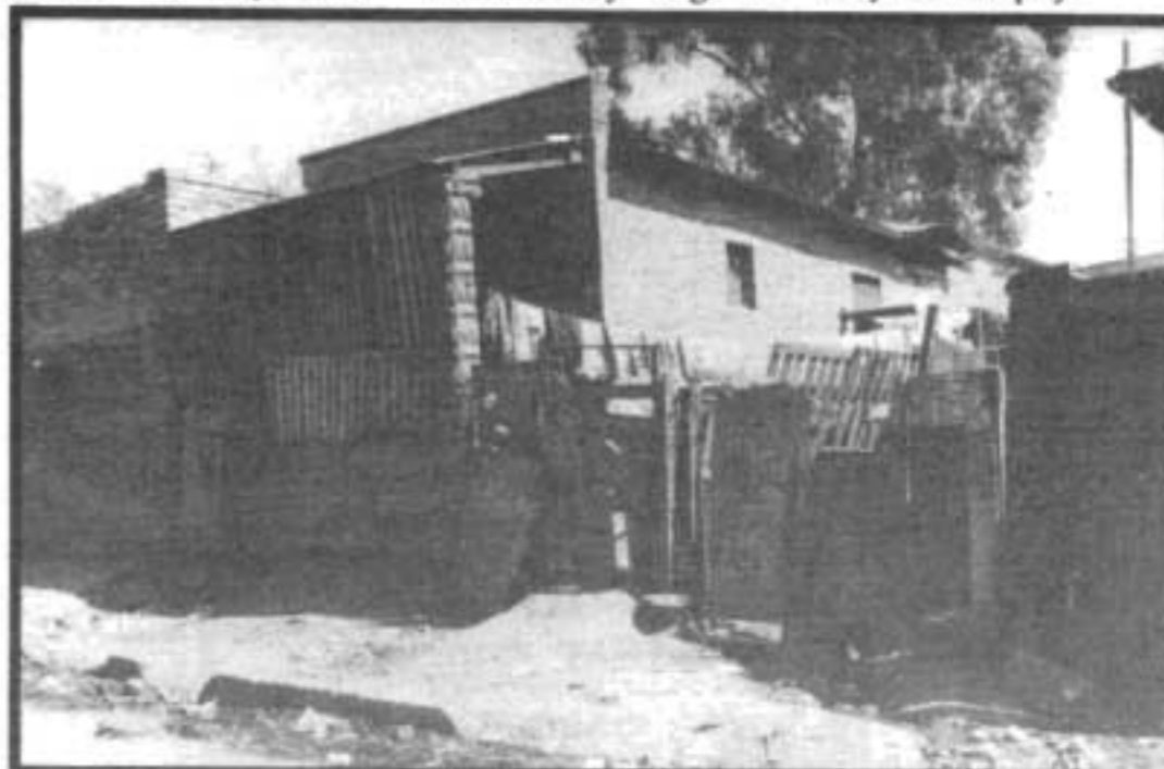
Old homes in Alexandra township were broken down to make way for new houses at high rentals
