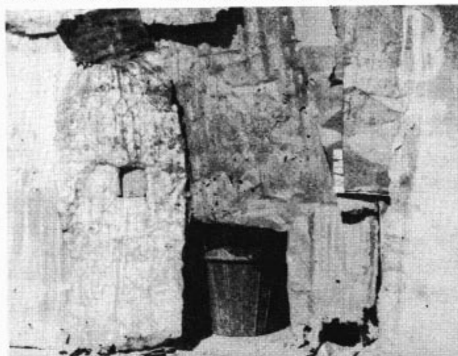
Thousands of Cape Flats residents still use bucket toilets.
