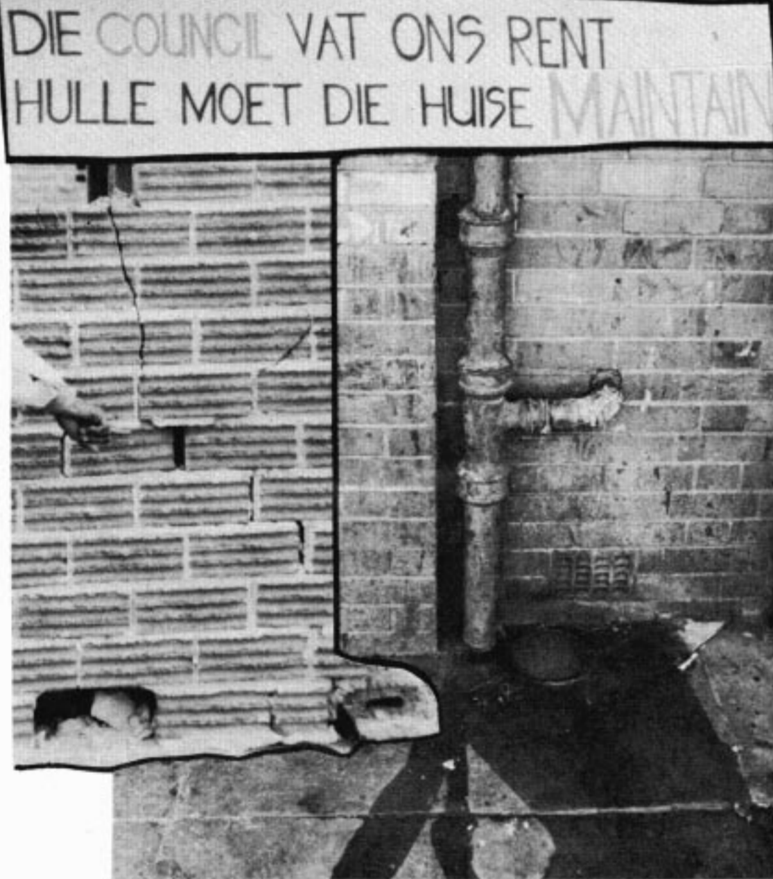
CAHAC rallies communities around housing problems.
