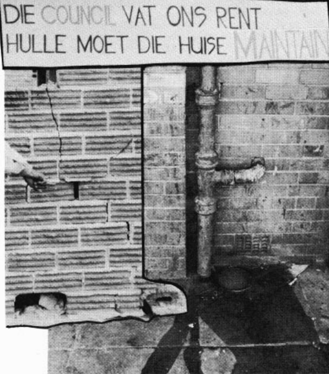
CAHAC rallies communities around housing problems.
